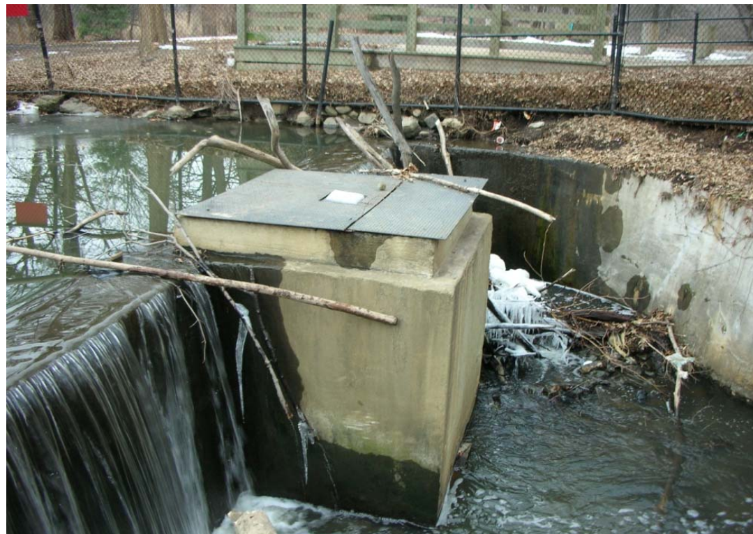
Overflow weir structure
