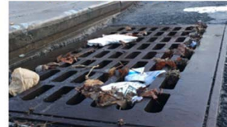
■ Catch Basin Hooding
