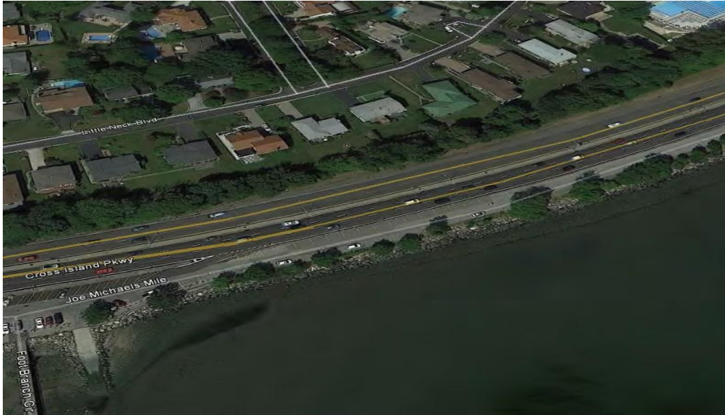
Figure 2-18. Western Shoreline of Little Neck Bay Near 27th Ave. (Looking West)
