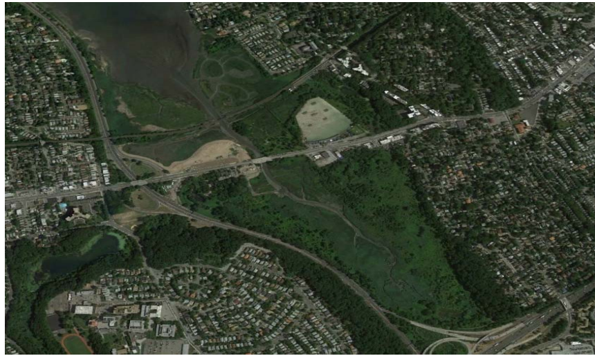
Figure 2-17. Shoreline of Alley Creek (Looking North)
