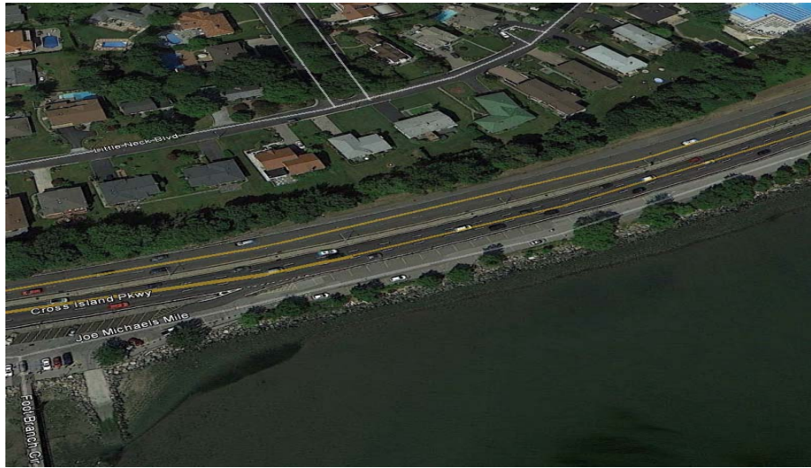
Figure 2-15. Western Shoreline of Little Neck Bay Near 27 th Ave. (Looking West)
