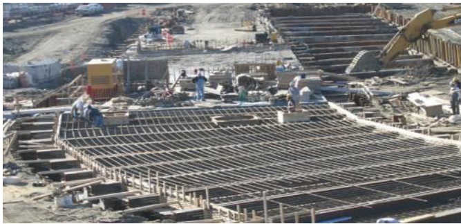
CSO Storage Facility
