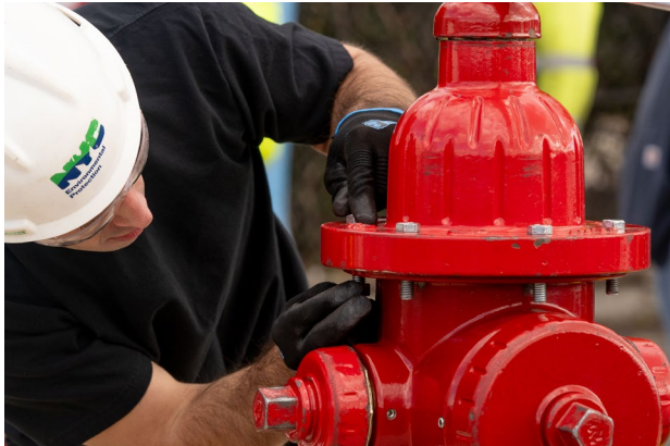
DEP employee performing hydrant maintenance.
