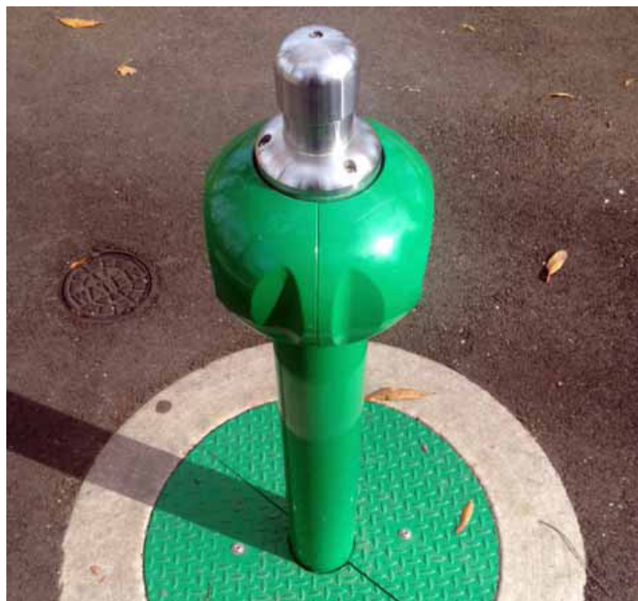
Figure 5: Retrofitted Lindower Park Spray Shower Bollard
