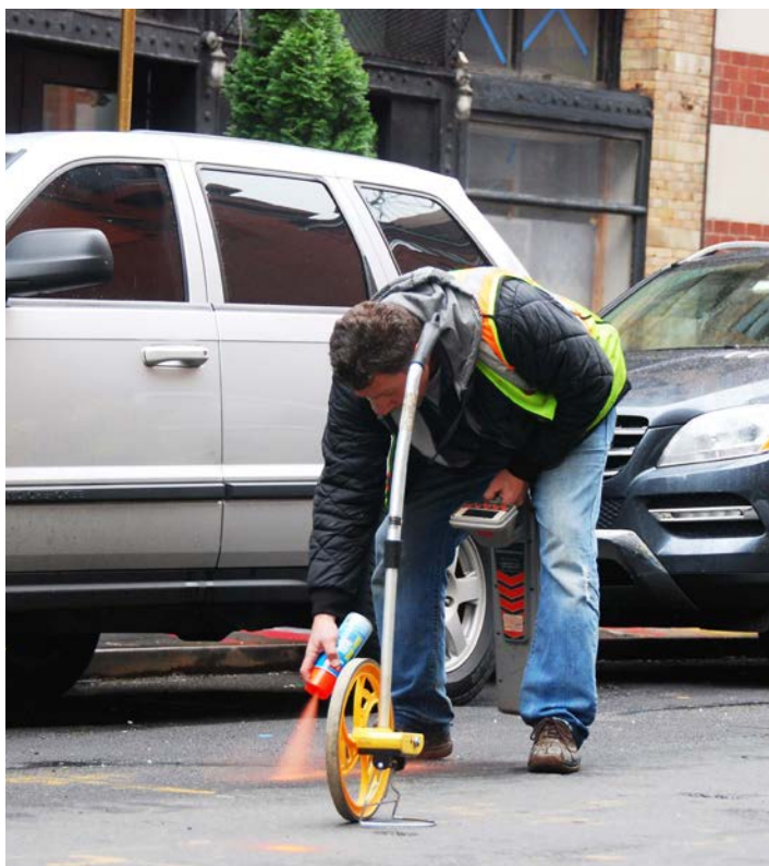
Figure 14: Leak location being marked
