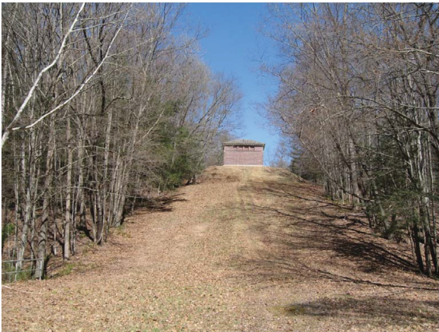
Photograph 2: Tongore North Siphon Chamber.
