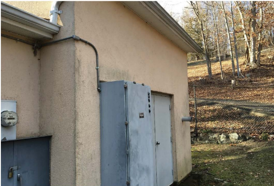
Photograph 2: View of the eastern facade of the structure housing the New Paltz Pump Station. Photograph taken facing west.
