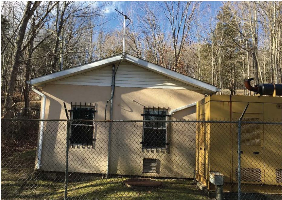
Photograph 1: View of the southern facade of structure housing the New Paltz Pump Station. Photograph taken facing northwest.
