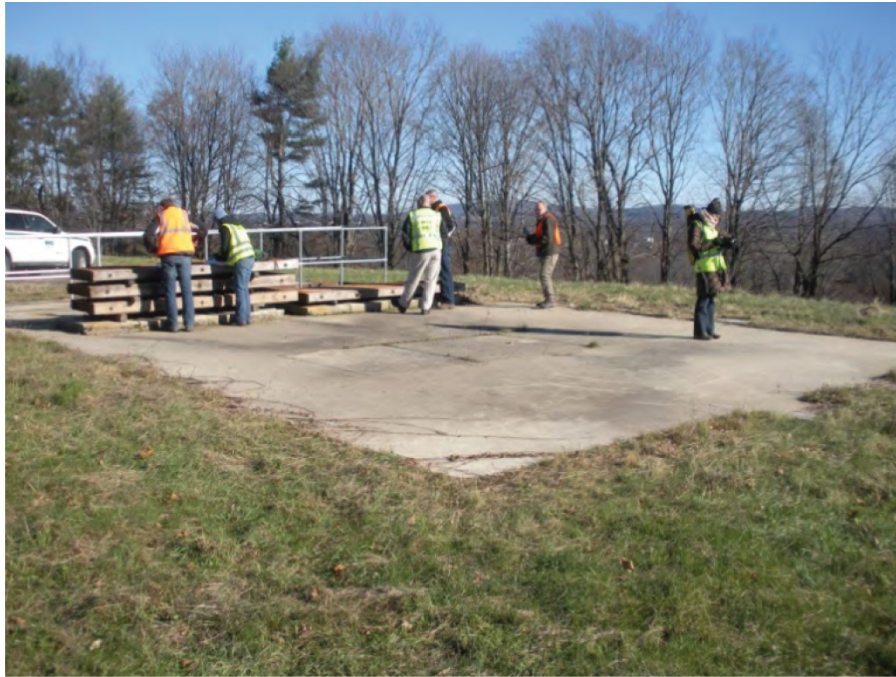
Photograph 1: Wallkill Downtake Chamber looking northeast.
