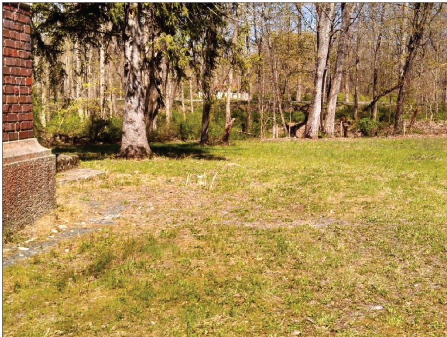
Photograph 2: View looking north from Rondout Drainage Chamber superstructure. The weir chamber is in front of the large evergreen tree.
