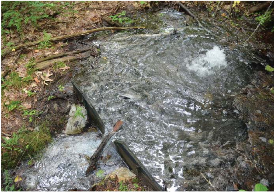
Photograph 3: Leak 4 flows through weir.
