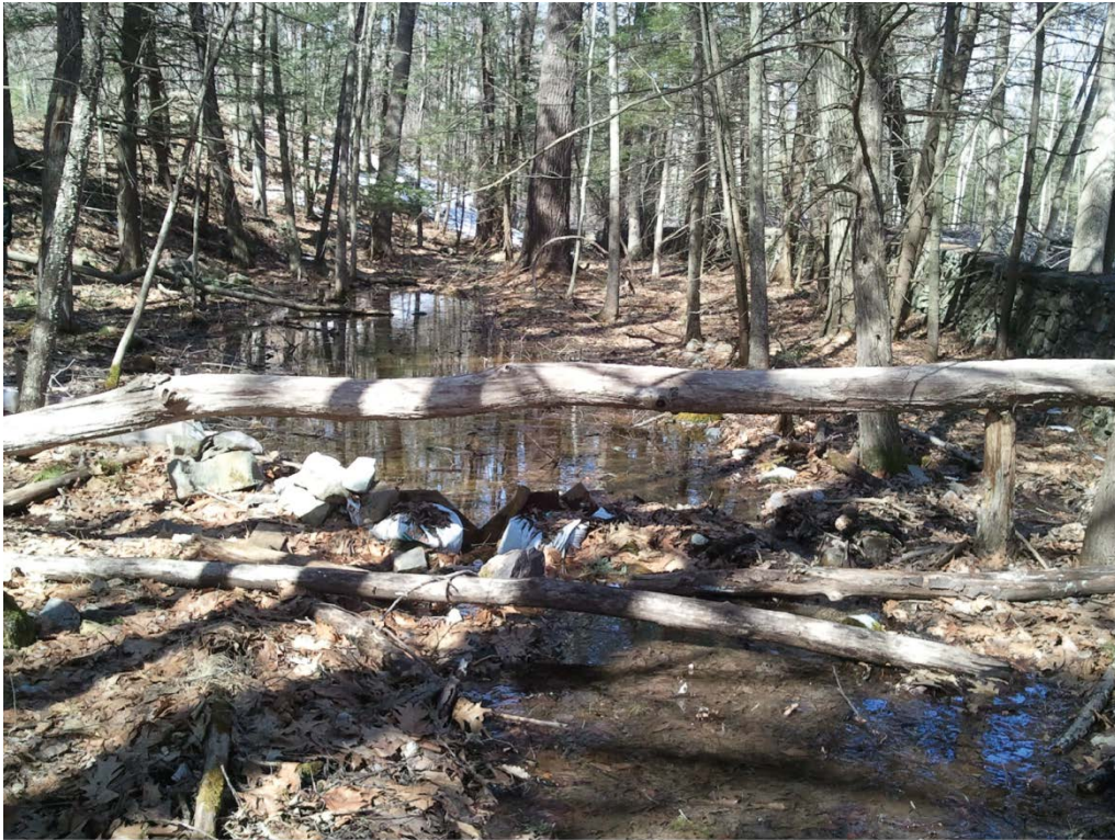
Photograph 3: Ponded area at Leak 2 flowing towards the weir. Photograph taken facing north.
