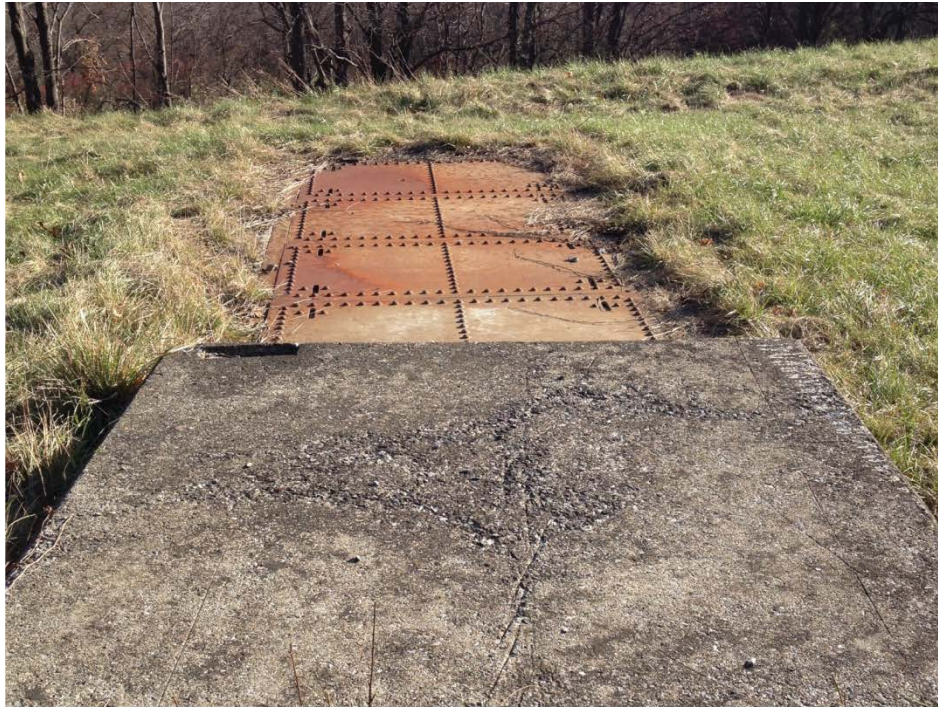
Photograph 3: View of existing boathole from the ground surface.
