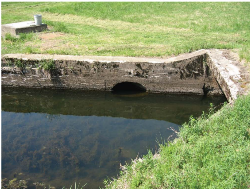
Photograph 2: Washington Square, Steel Pipe Siphon west blow-off chamber discharge pipe to Silver Stream; looking west.
