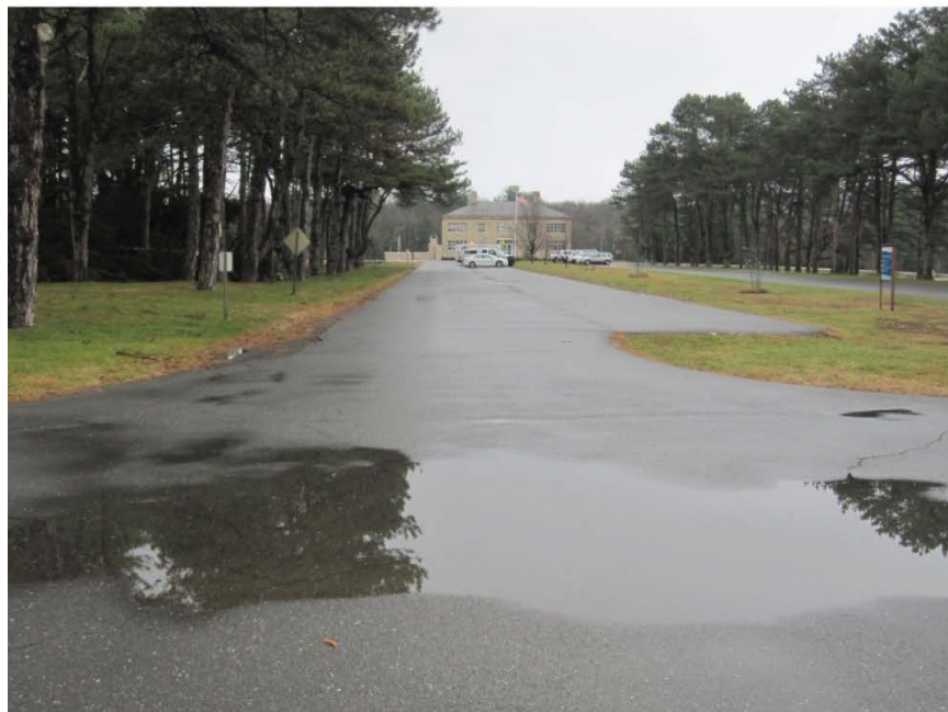
Photograph 2: Access driveway to the screen chamber site. Taken looking southeast at the Ben Nesin Laboratory.
