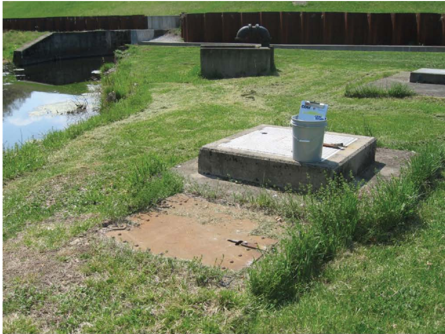
Photograph 1: Washington Square, Steel Pipe Siphon west blow-off chamber exterior, valve vault, manway, and vent; looking southwest.
