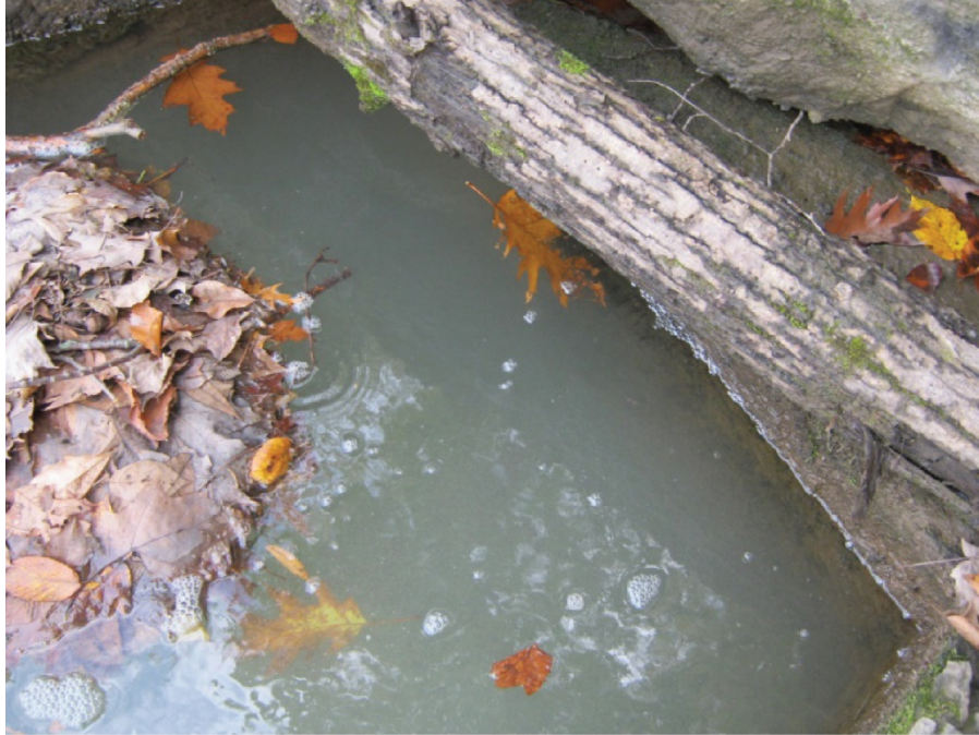
Photograph 1: View of Leak 5 at Rondout Creek, with bubbles indicating the location of the submerged conduit pipe. Concrete headwall is visible in the upper right-hand corner.
