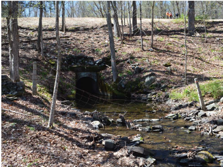
Photograph 2: Hendricks Killitje flowing through the culvert under the Catskill Aqueduct. Approximate location of the temporary stream crossing, upstream of the confluence with Leaks 1A and 1B.
