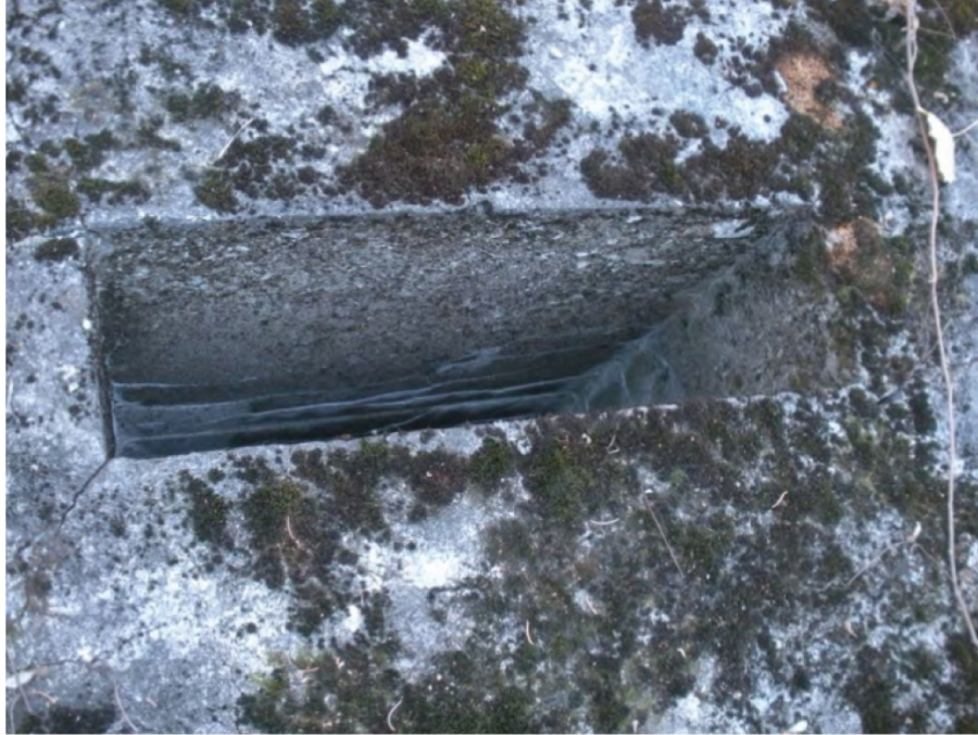
Photograph 1: Rondout Uptake Chamber ground opening.
