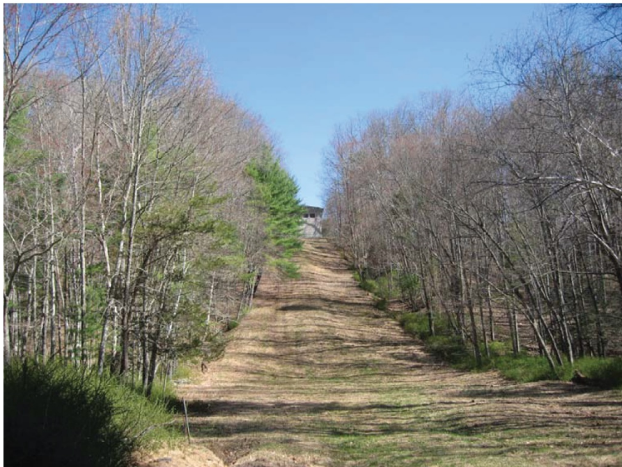
Photograph 2: Looking north toward North Siphon Chamber from siphon blow-off chambers.
