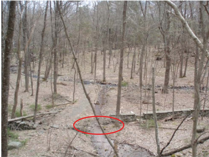
Photograph 1: Leaks 1A and 1B merge near the rock boundary wall (red circle) and flow into Hendricks Killitje, a tributary of the lower Esopus Creek, visible in the background. Photograph facing east.
