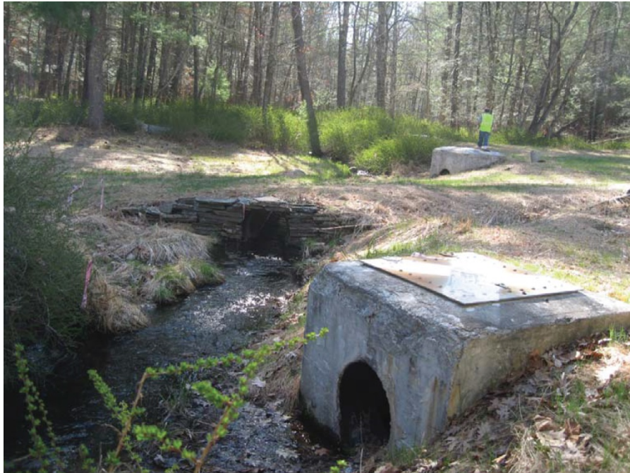
Photograph 1: West and middle siphon blow-off chambers in the relic channel of Esopus Creek. Existing stream crossing located between the two blow-off chambers.
