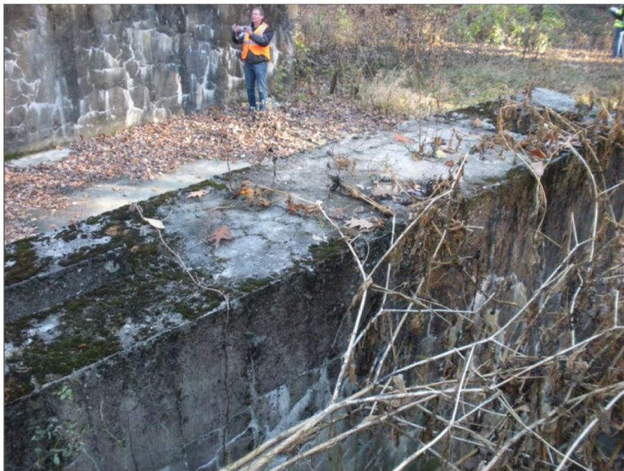
Photograph 2: Rondout Uptake Chamber looking southeast.
