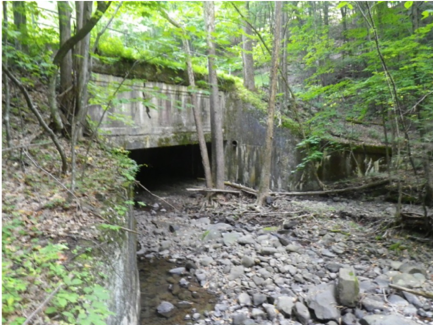
Photograph 1: Grass-covered Tongore Bridge over Tongore Creek, looking east.
