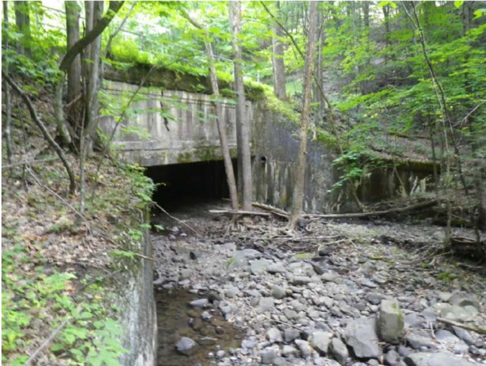
Typical Siphon Bridge Structure
