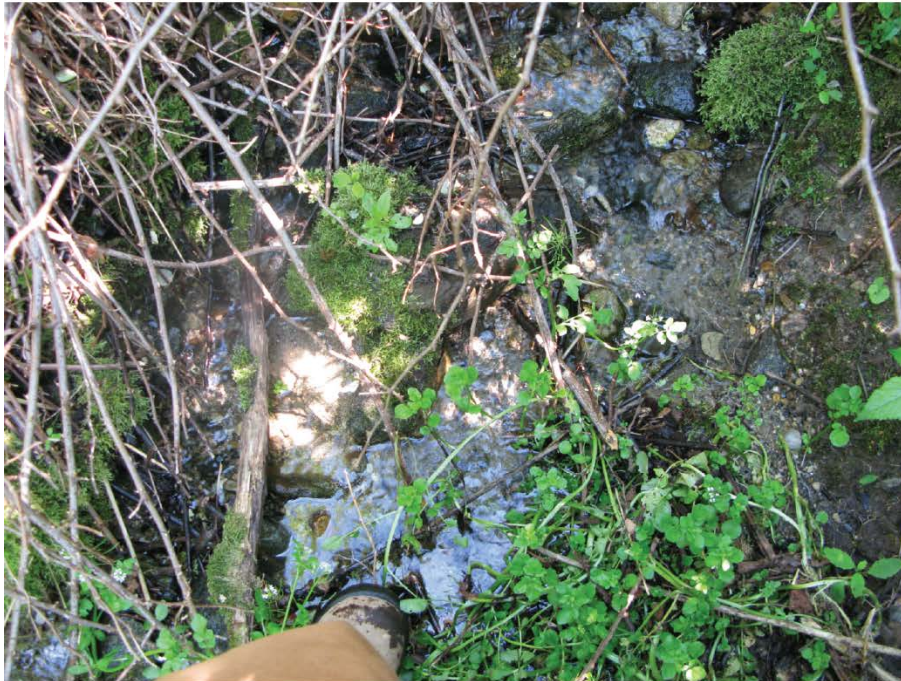
Photograph 4: Leak 9 with shallow water depths as it flows north along aqueduct. Photograph taken facing upstream (south).
