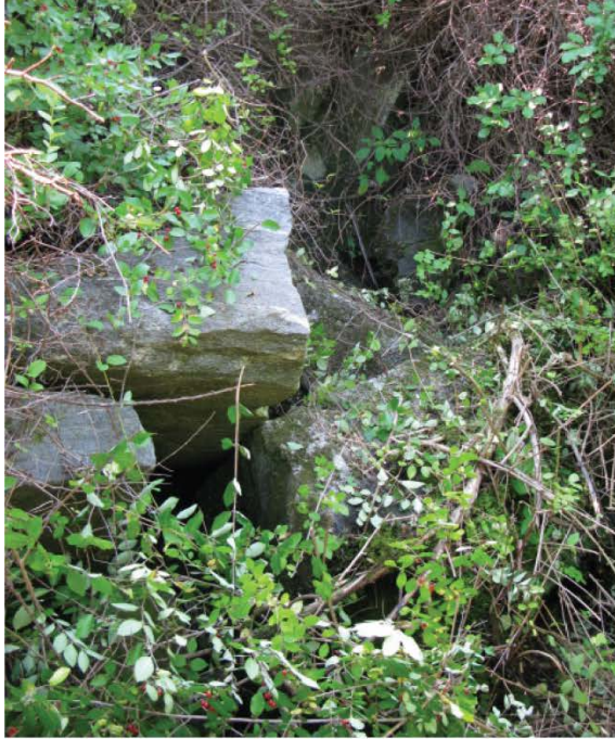
Photograph 3: Riprap at the base of the aqueduct berm. Leak 9 originates from the riprap. Photograph taken facing southeast.
