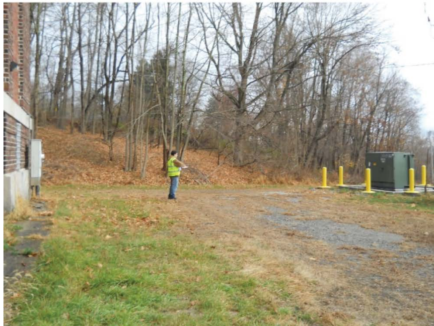
Photograph 2: Croton Lake Downtake Chamber looking east at the existing access road and potential staging area.
