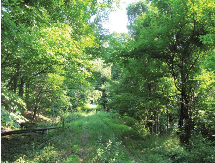
Photograph 1: View of the aqueduct right-of-way looking north.
