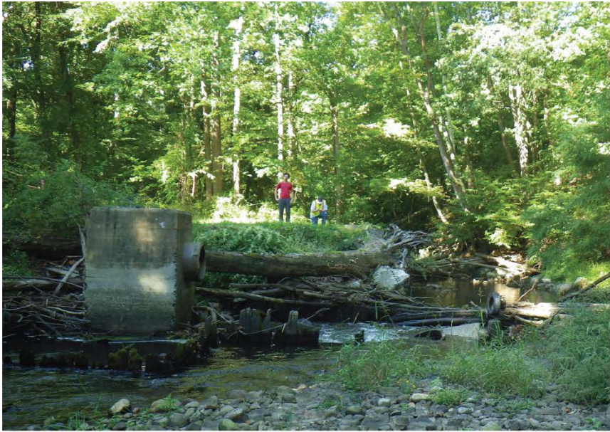
Photograph 1: Peekskill Hollow Creek with exposed blow-off chamber.
