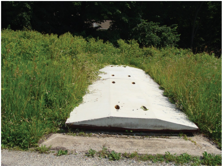
Photograph 1: Pleasantville Cut-and-Cover Tunnel boathole.
