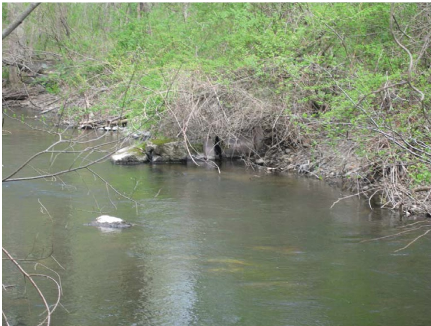
Photograph 2: Sprout Brook Steel Pipe Siphon Blow-Off Chamber. Note the exposed chamber in the channel.
