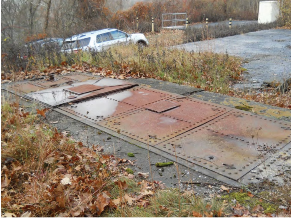
Photograph 3: Croton Lake Pressure Tunnel Uptake Chamber (facing northwest).
