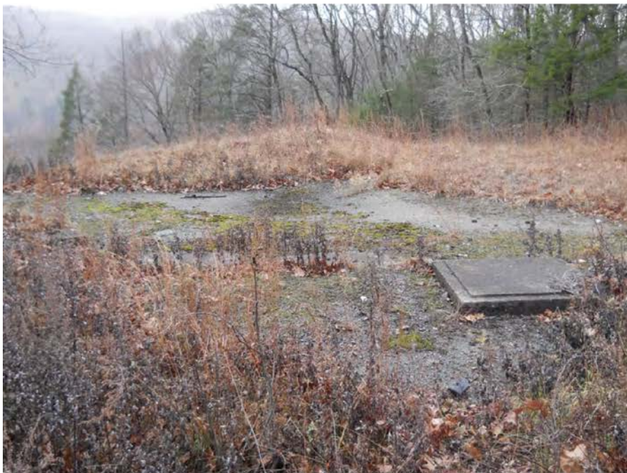
Photograph 2: Croton Cut-and-Cover Tunnel Boathole (facing northeast).
