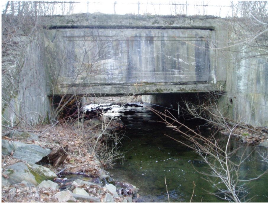
Photograph 1: Foundry Brook Bridge.
