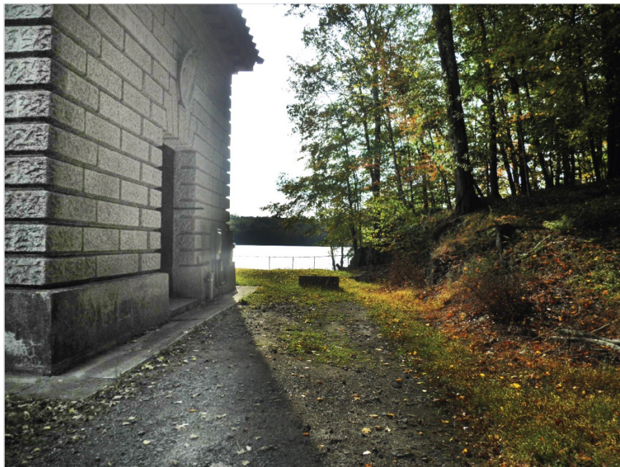
Photograph 2: Staging area adjacent to Catskill Influent Chamber (looking south).
