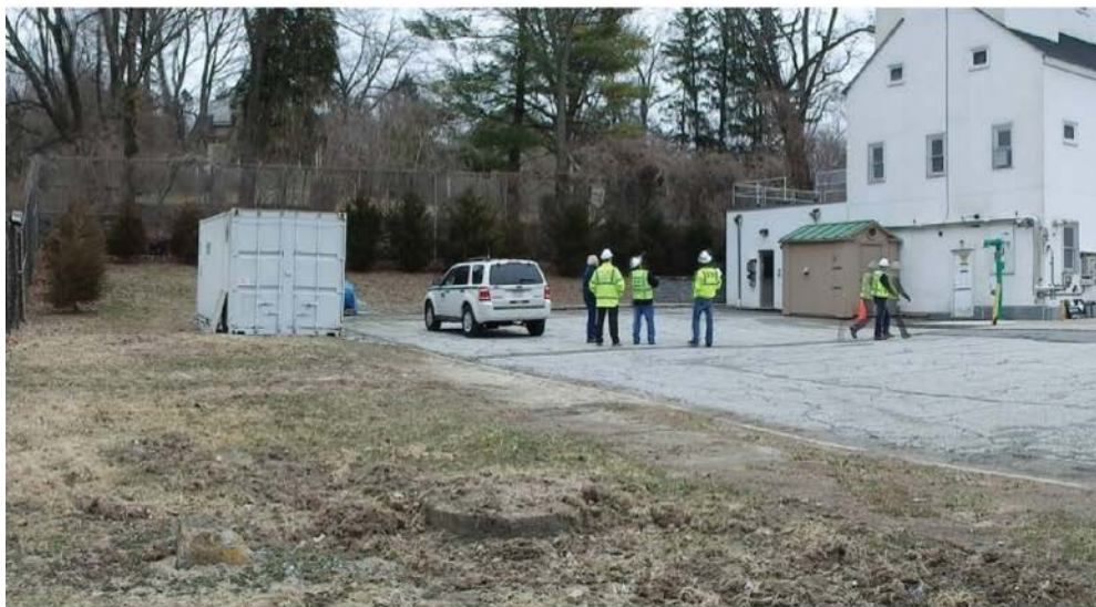
Photograph 2: Location of proposed dechlorination facility adjacent to the existing Alum Plant looking southwest.
