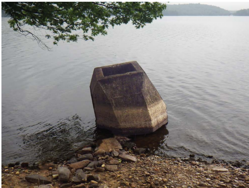
Photograph 1: View of access manhole to Catskill Kensico Bypass Tunnel that is off-shore in Kensico Reservoir. The manhole would be abandoned.
