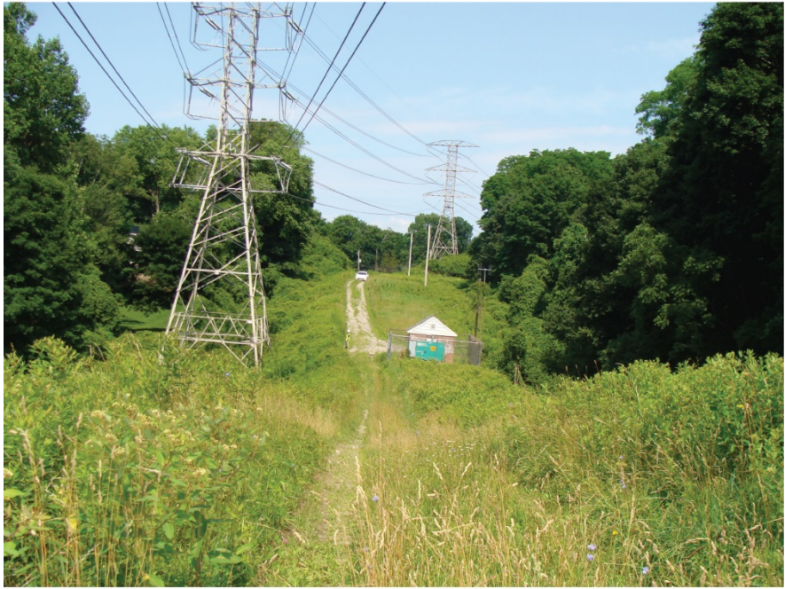
Photograph 2: Pleasantville Cut-and-Cover Tunnel boathole, looking northwest along access road.
