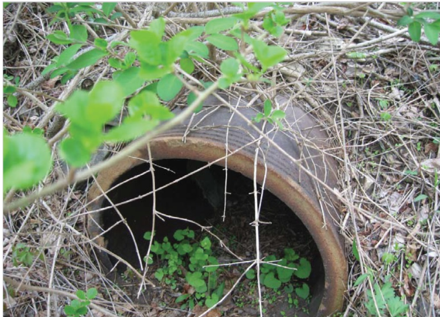
Photograph 2: Harlem Railroad Steel Pipe Siphon Blow-off Chamber discharge pipe shown containing sediment.
