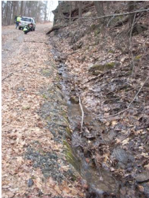
Photograph 1: Flowpath of Leak 7 along DEP Access Road (looking northward).
