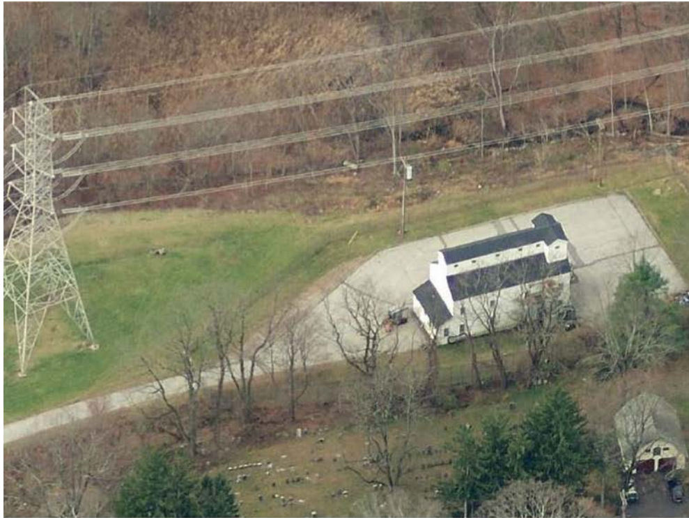
Photograph 1: Aerial view of the Pleasantville Alum Plant facing west.
