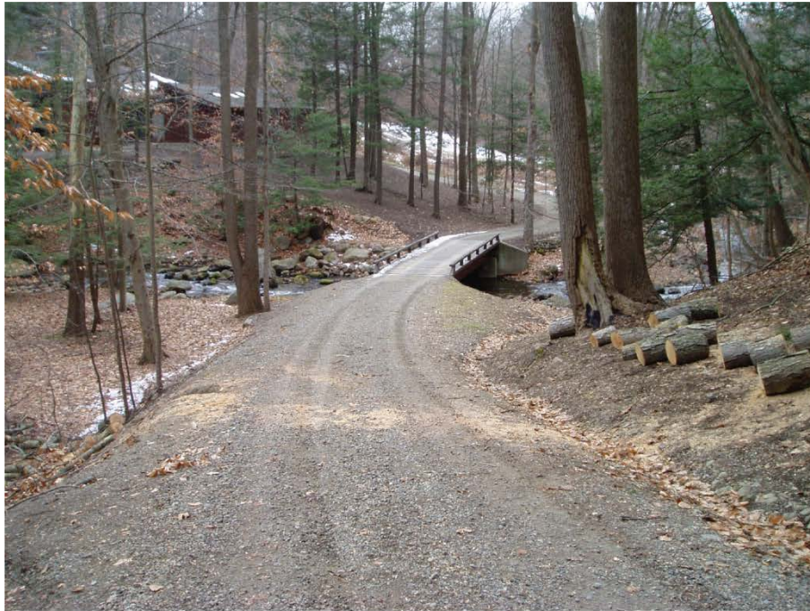
Photograph 1: Access bridge on private driveway to Indian Brook Bridge and Blow-off Chambers.
