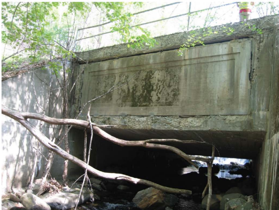
Photograph 2: Indian Brook Bridge.
