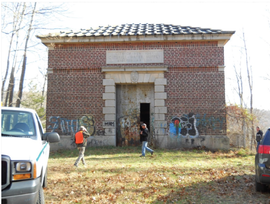
Photograph 2: Looking south from the Sprout Brook Steel Pipe Siphon North Chamber from the location of the new boathole.
