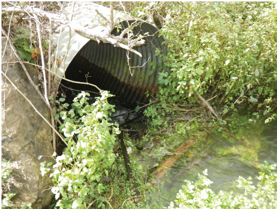
Photograph 9: View south at culvert in the middle of Stream Segment 3
