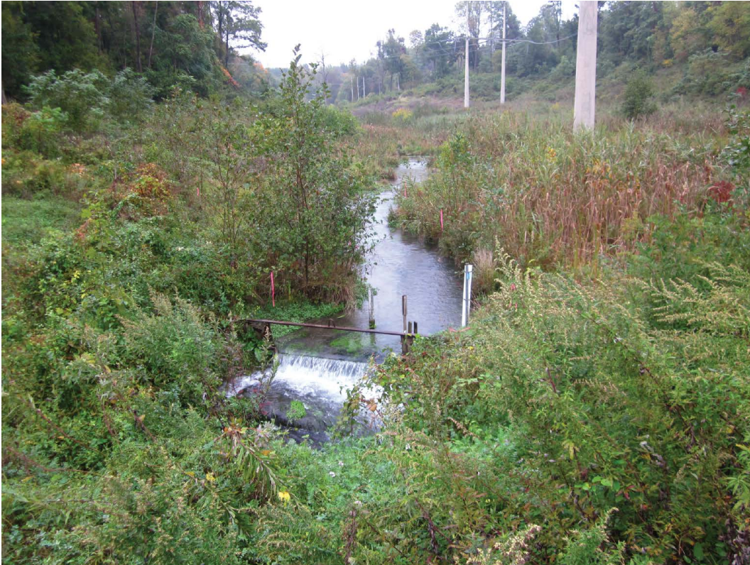
Photograph 23: View north towards weir (center bottom), adjacent to intersection of River and Danskammer Roads
