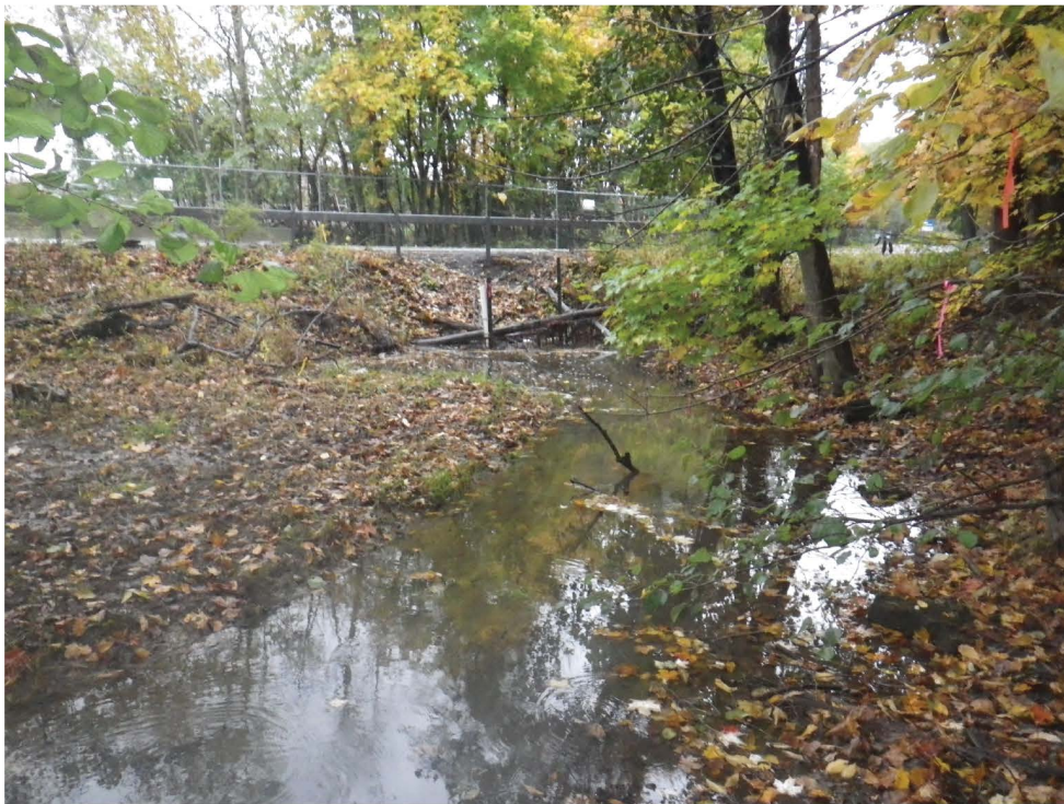
Photograph 5: View south at culvert under River Road, at downstream end of Stream Segment 2
