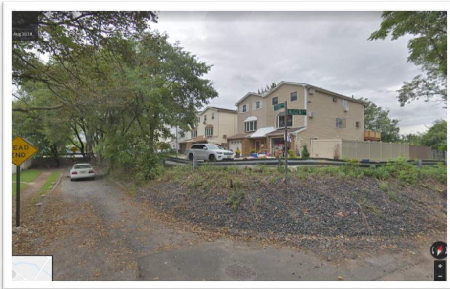
Inset 3. Unimproved segment of Stobe Avenue, intersection of Nugent Avenue, showing the rubble embankment and guard rail. The higher segment of Stobe is just beyond the guard rail. Google Street View image, August 2018.
