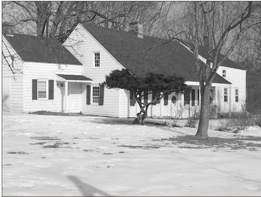
View of Hammond House looking northeast 1
