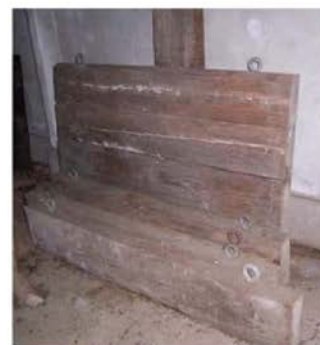
Partial Stop Shutter Assembly shown Above-Grade
