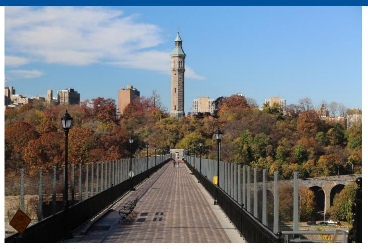
The 41-mile Old Croton Aqueduct was the first to deliver a clean and plentiful supply of water to New York City. The High Bridge, completed in 1848 and hailed as an engineering masterpiece, carried the aqueduct across the Harlem River on large stone arches.
