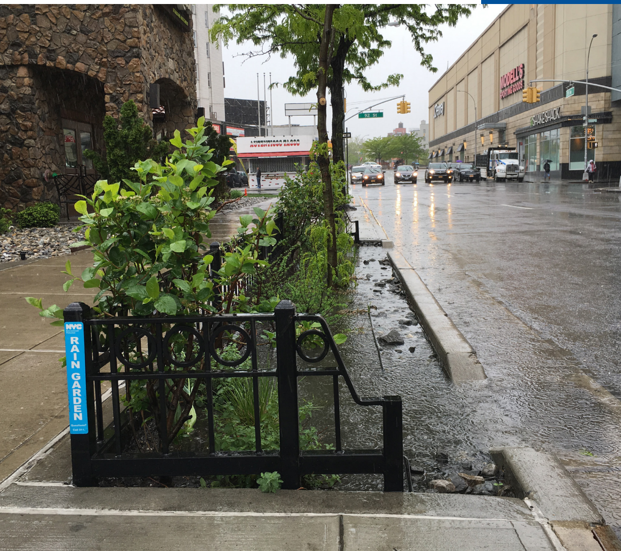
Rain gardens intercept stormwater before it enters the sewers, allowing it to infiltrate into the ground below.
