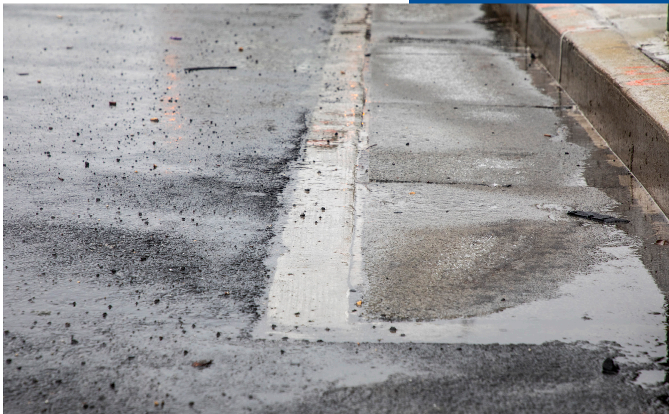
Pre-cast porous panels can be sited in the roadway, unlocking additional areas to absorb stormwater.
