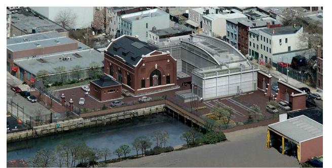
In December 2013, DEP completed a rehabilitation of the 1.3 mile Gowanus Canal Flushing Tunnel, which brings oxygenated water from New York Harbor to the head of the canal.
