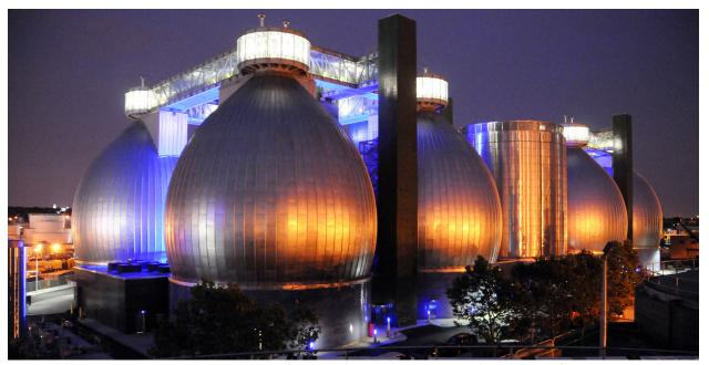
In 2013, DEP announced a partnership with National Grid to purify anaerobic digester gas from Newtown Creek Wastewater Treatment Plant and inject it into the natural gas grid, which will allow the plant to beneficially use 100% of the gas it produces.
