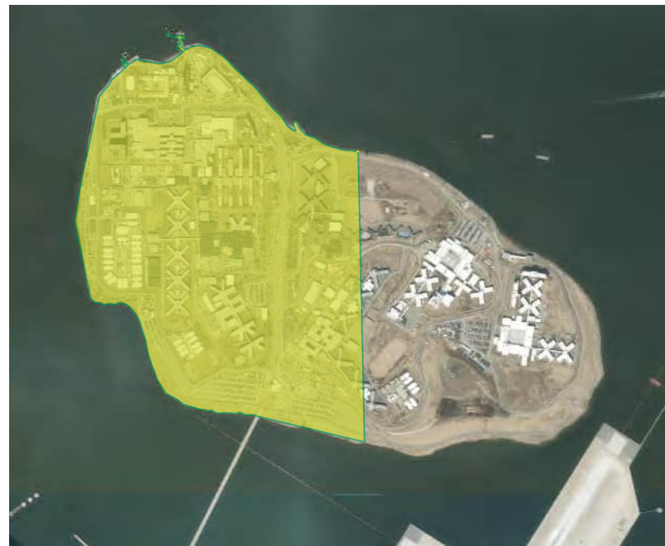
Aerial view of the estimated area of a new WRRF on Rikers Island. (Courtesy of Esri)
