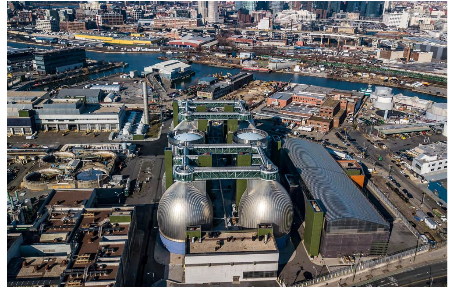
DEP's wastewater infrastructure is critical to protecting public health and the environment. The Newtown Creek WRRF is one of 14 in the New York City system. (Courtesy of NYCDEP)
