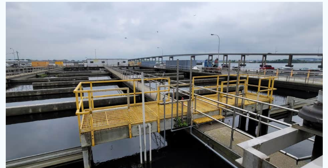
The Rikers Island bridge can be seen beyond the disinfection tanks at the Bowery Bay WRRF. (Courtesy of NYCDEP)
