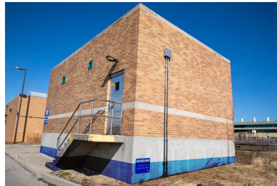
Ten WRRFs and more than 40 wastewater pumping stations were affected by Superstorm Sandy in 2012. This image shows the High Water Mark from Superstorm Sandy at the at the Hunts Point WRRF, in blue, demonstrating that most of the tanks were submerged and unable to maintain treatment. In addition, much of the equipment and materials below ground – of which there are many – were heavily damaged. (Courtesy of NYCDEP)
