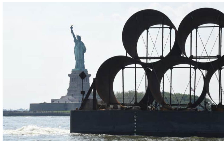
DEP is always working to improve New York City's water infrastructure, from our water supply system to our wastewater treatment operations. These steel pipe liners are part of a major project to re-enforce the water supply system so we can continue providing New Yorkers with excellent water services for generations to come. (Courtesy of NYCDEP)
