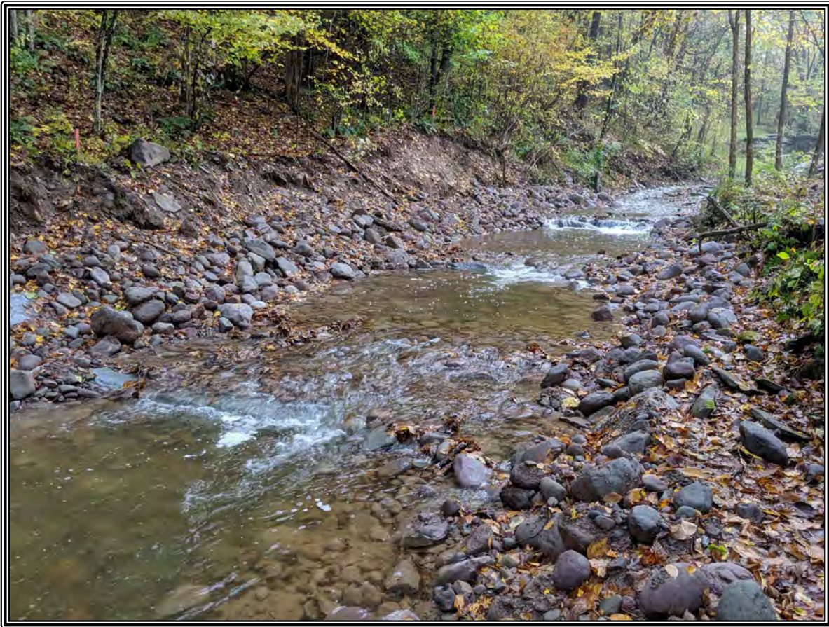
Marvin Hollow Grade Control Town of Walton, NY constructed in 2019
