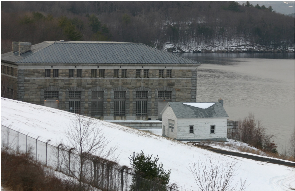
Figure 3.23 Rondout Reservoir Effluent Chamber. Photo by Chris Nadareski
