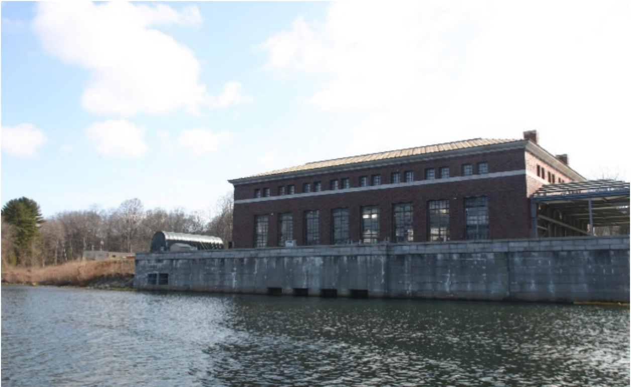
Figure 3.21. West Branch DEL10 Effluent facility. Photo by Chris Nadareski.
