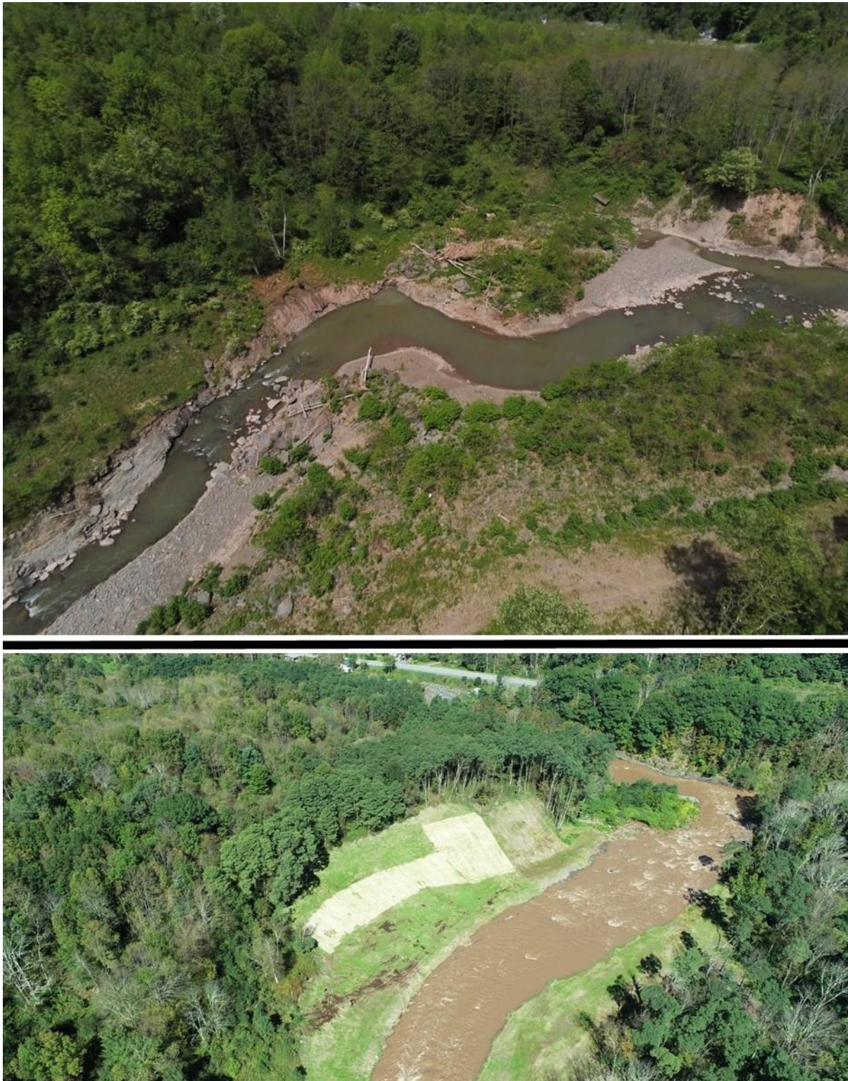
Figure 4.7 Red Falls Project Phase 2 prior to restoration (top) and Phase 2 following restoration (bottom).
