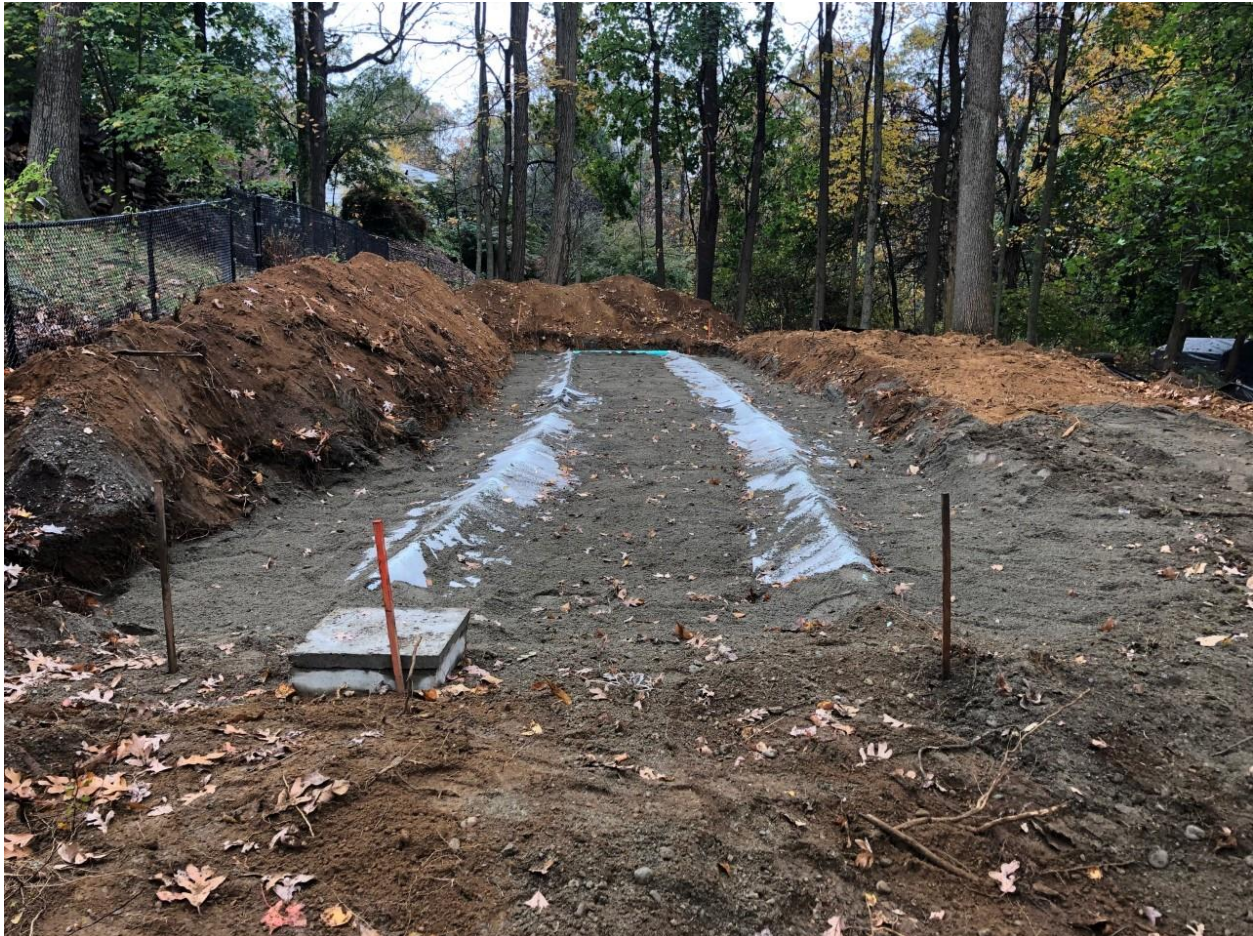
Figure 4.19 Installation of Eljen system for septic repair near Kensico Reservoir.
