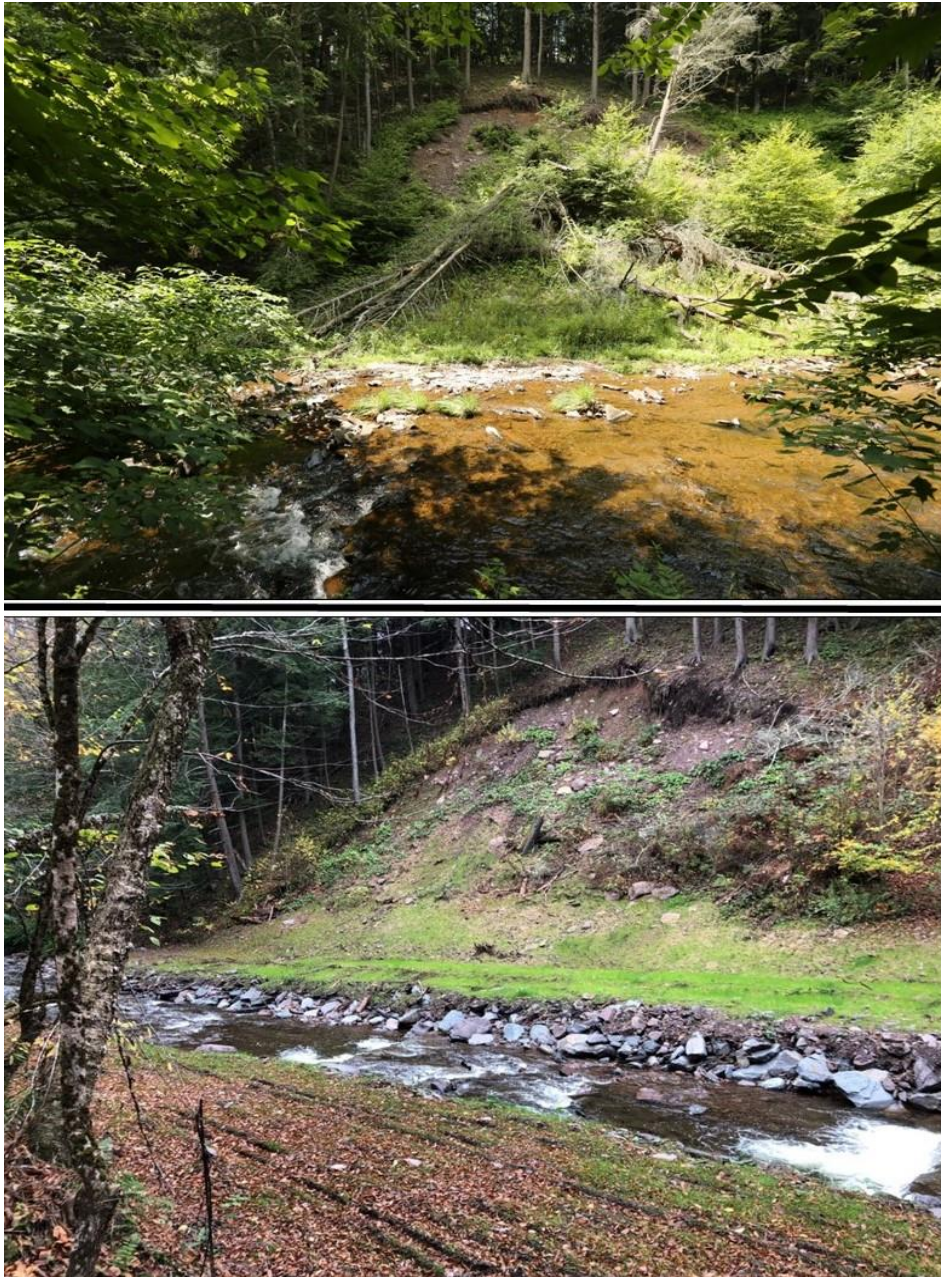
Figure 4.10 Steele Brook at Reservoir Park before (top) and after (bottom) construction.
