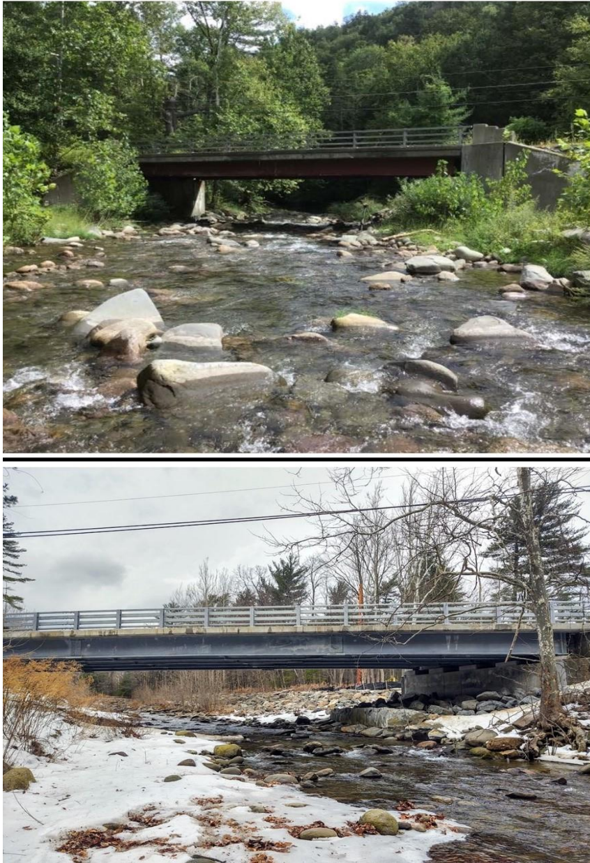
Figure 4.9 Maltby Hollow Bridge: Top is before replacement; bottom is after replacement.
