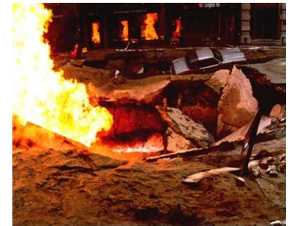
Watermain break, street collapse, gas pipeline cut, and fire occurred.
