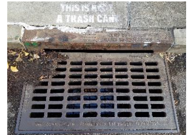
Catch basins, leading to the underground, NYC
