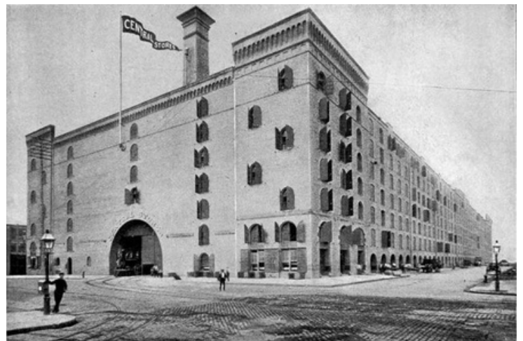
Figure 15. Warehouse, Heavy Timber Framing (Lamont-Doherty Earth Observatory, 2021)
