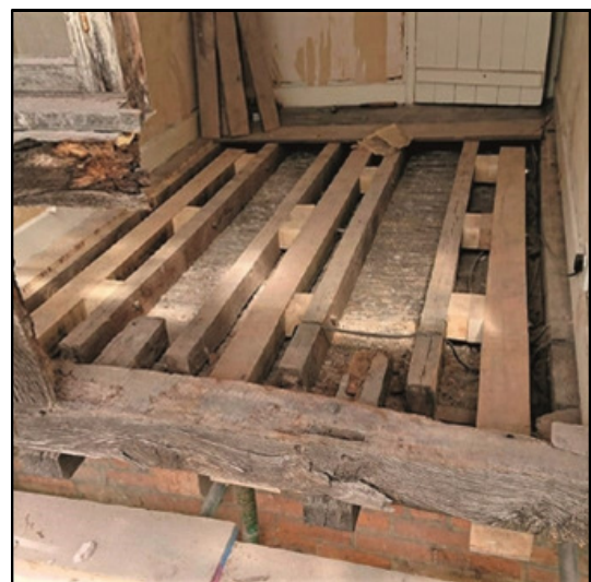
Figure 22. Example of Old-growth Wood Joist
