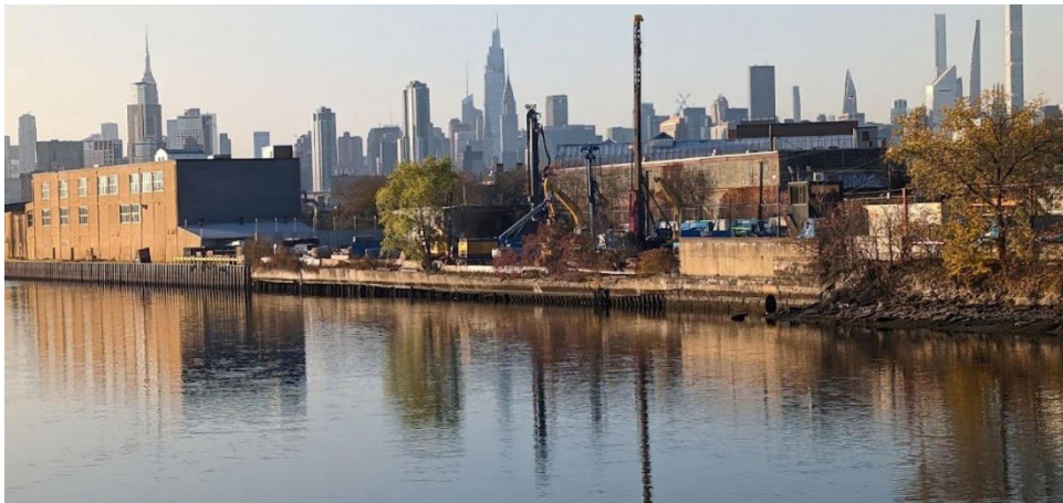
Figure 1. Urban Industries bordering Newtown Creek and Manhattan Skyline beyond. CCNY MUPUD Studio 2023.
