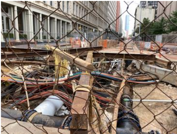
40 Worth Street, NYC, roadway reconstruction project, November 2021.
