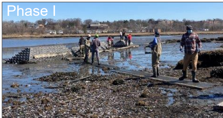
Oyster castle installation with staff and volunteers – March 2021
