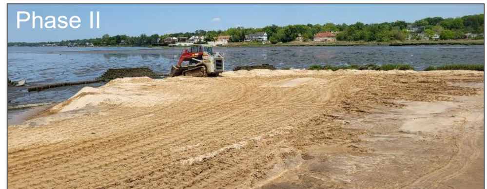
Sand placement on mudflat using front loader – May 2023
