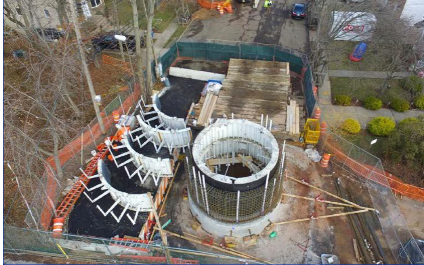
Constructing Caisson sections approximately 20' diameter and approximately 20' high
