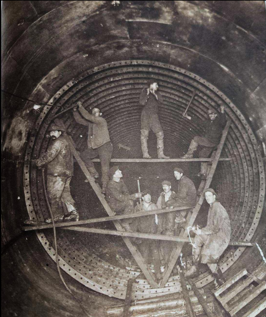
Sand Hogs Removing Liner Plates
