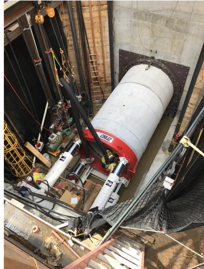
Jacking concrete pipe
