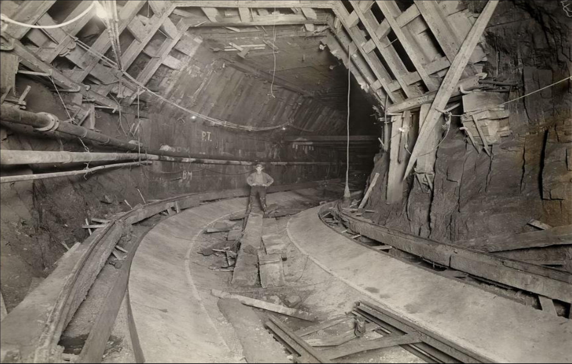
City Tunnel #2 Construction, just South of Hillview Reservoir (May 24th, 1932)
