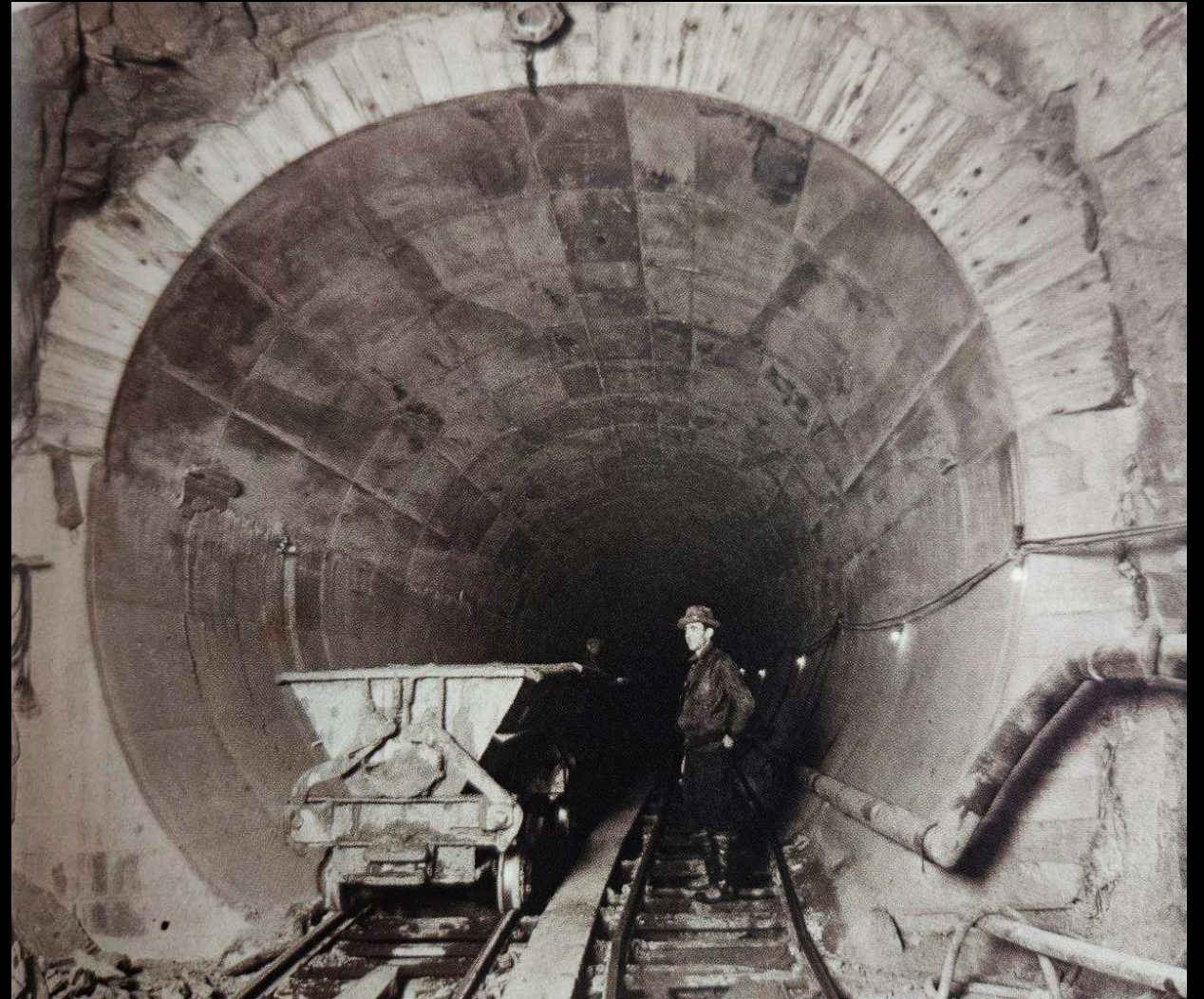
Liner Plates Removed
