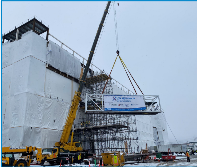
Lifting Frame To Temporary Platform For Subfab Access
