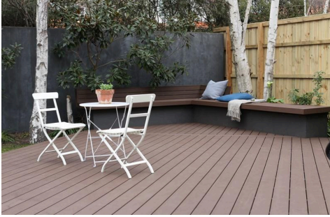
Figure 5: Outdoor deck/landscaping with recycled plastic
