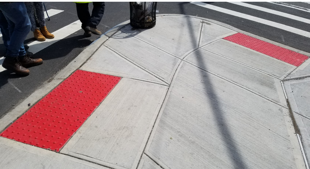
Detectable Warning Surfaces, Grand Avenue and Vanhorn / Seabury, Queens
