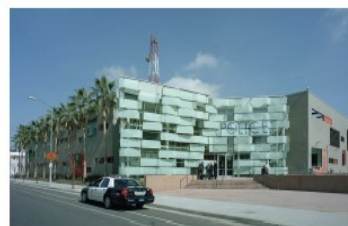
Hollenbeck Replacement Precinct, 2009 Los Angeles, California
