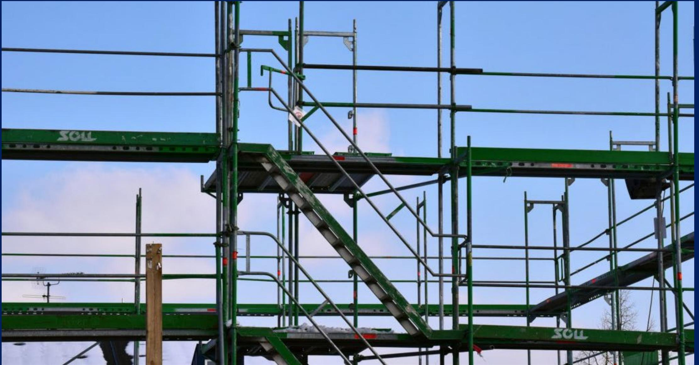
Each employee on a scaffold more than 10 feet above a lower level shall be protected from falling to that lower level (Subpart L)
