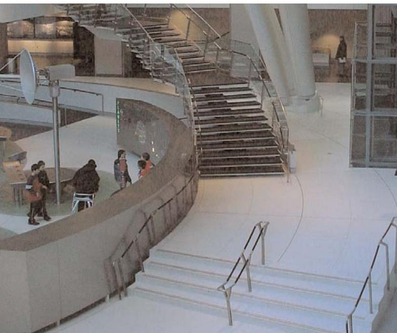
Many buildings have level changes beyond the allowable height. When an elevator is not a practical solution (e.g. change in level of a few inches), designers frequently use ramps or stairs to provide access to these areas. Even though the change in level may be slight, if not designed properly, people can find negotiating ramps and stairs difficult and dangerous.
