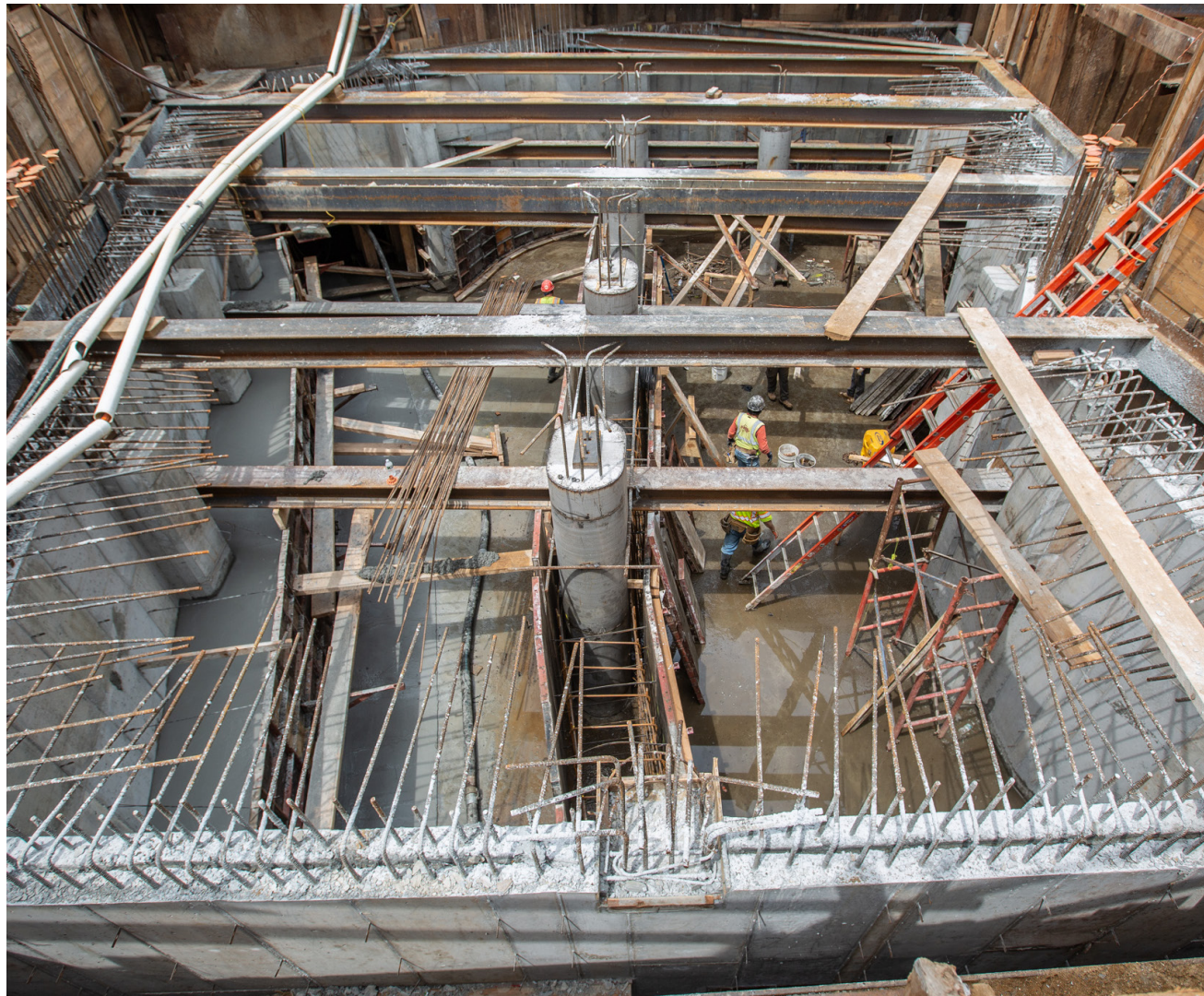
Sewer chamber construction underway on Jamaica Avenue, Southeast Queens
