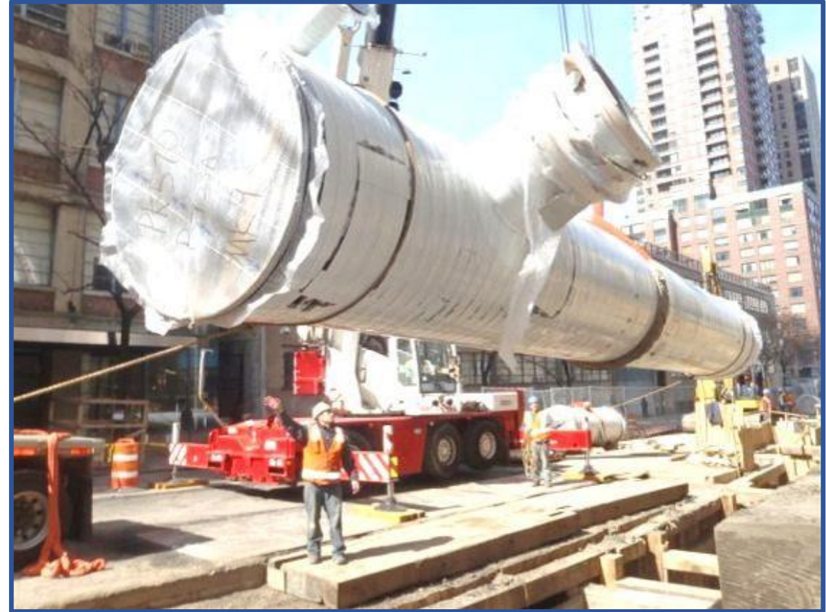
We Have To Make Room For 48" Pipes
