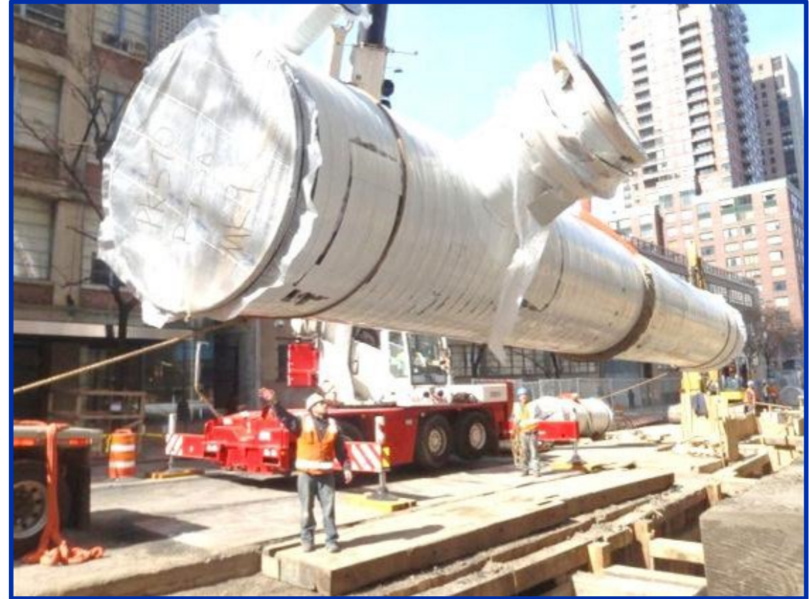
We Have To Make Room For 48" Pipes
