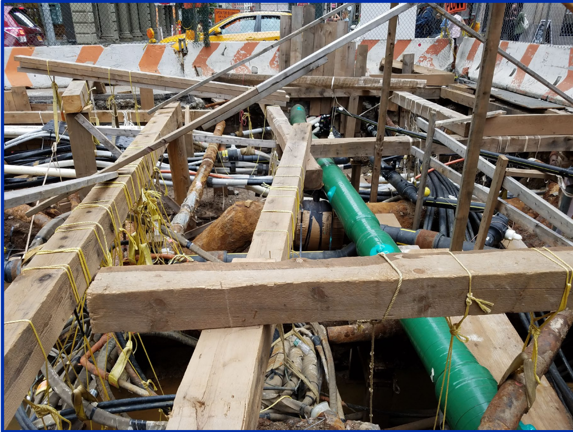
What It Looks Like Below the Roadway
