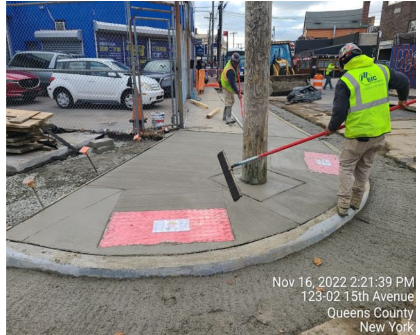
Construction of corner sidewalk and pedestrian ramp 15 th Avenue & 123 rd Street
