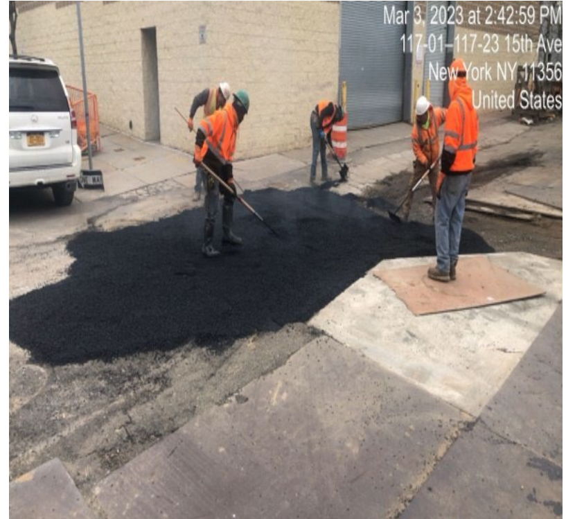
Backfill and asphalt around chamber 15 th Avenue & 117 th Street
