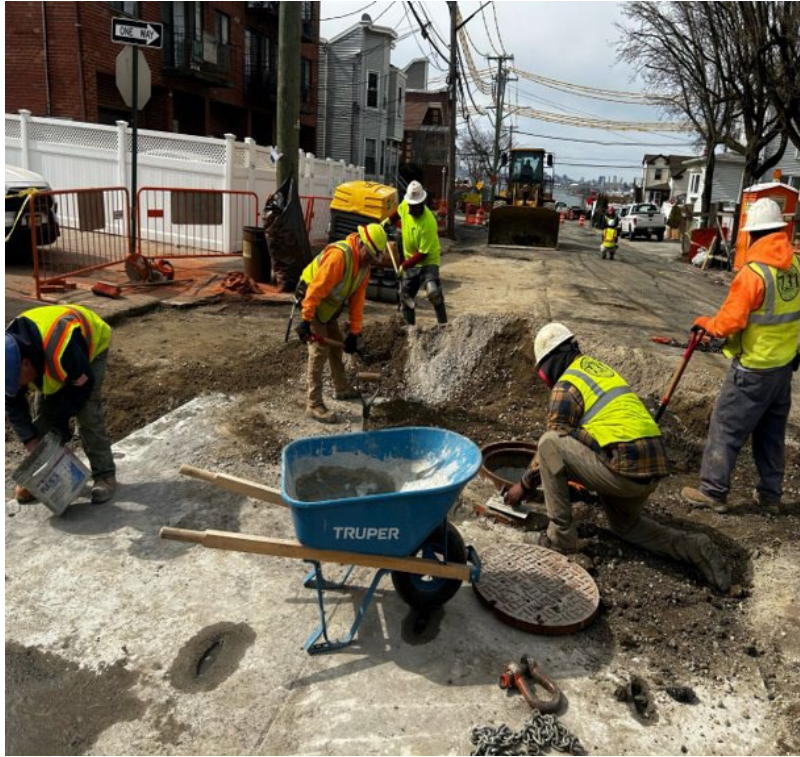
Chamber roof and casting installation 20 th Avenue
