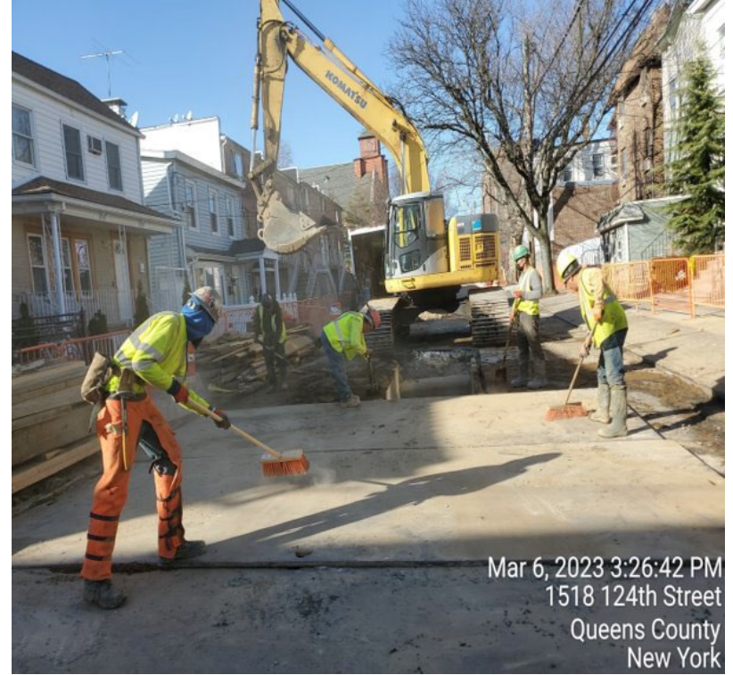
Cleaning on 124 th Street between 15 th & 18 th Avenues
