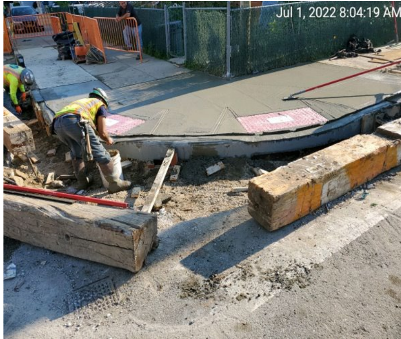
Construction of corner sidewalk and pedestrian ramp 14 th Avenue & 120 th Street
