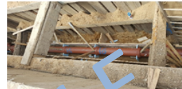
Installation of sanitary sewer on 119 th Ave.
