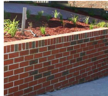
BRICK RETAINING WALL
