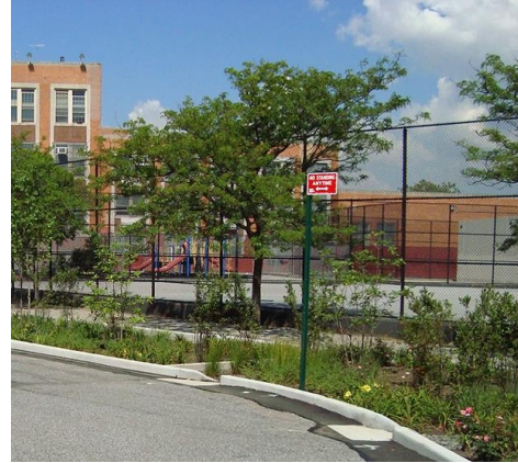
Stormwater Green Street Streets and sidewalks
