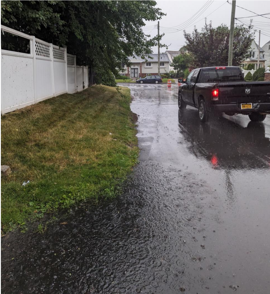
112TH AVE LOOKING SOUTH
