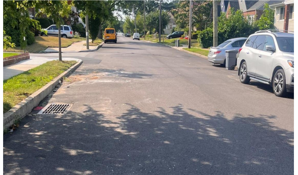
177TH ST LOOKING SOUTHEAST
