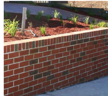
BRICK RETAINING WALL
