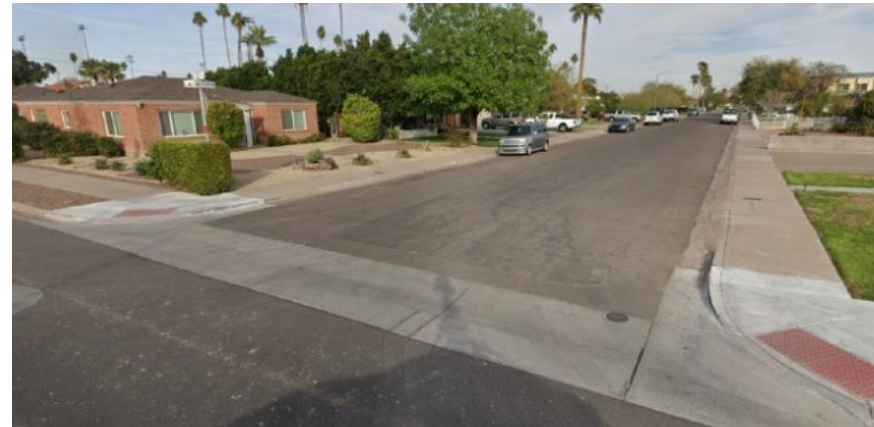
Depressed Gutter Gutter across intersections
