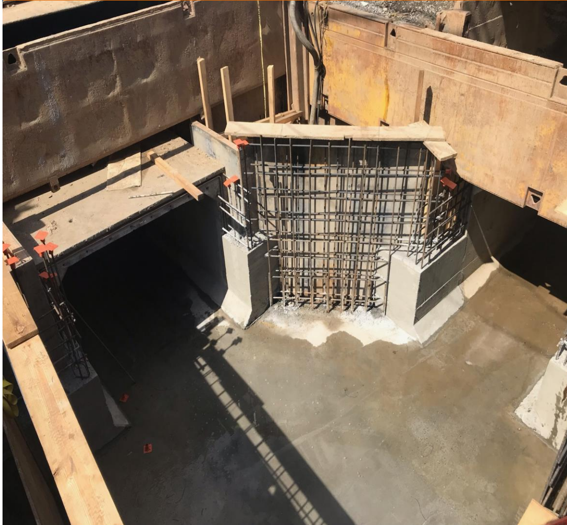
Chamber No. 3 Intersection of 15 th Avenue and 119 th Street
