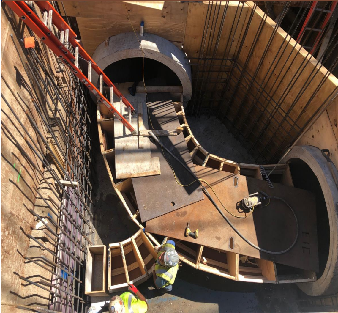
Chamber No. 6 Intersection of 20 th Avenue and 119 th Street
