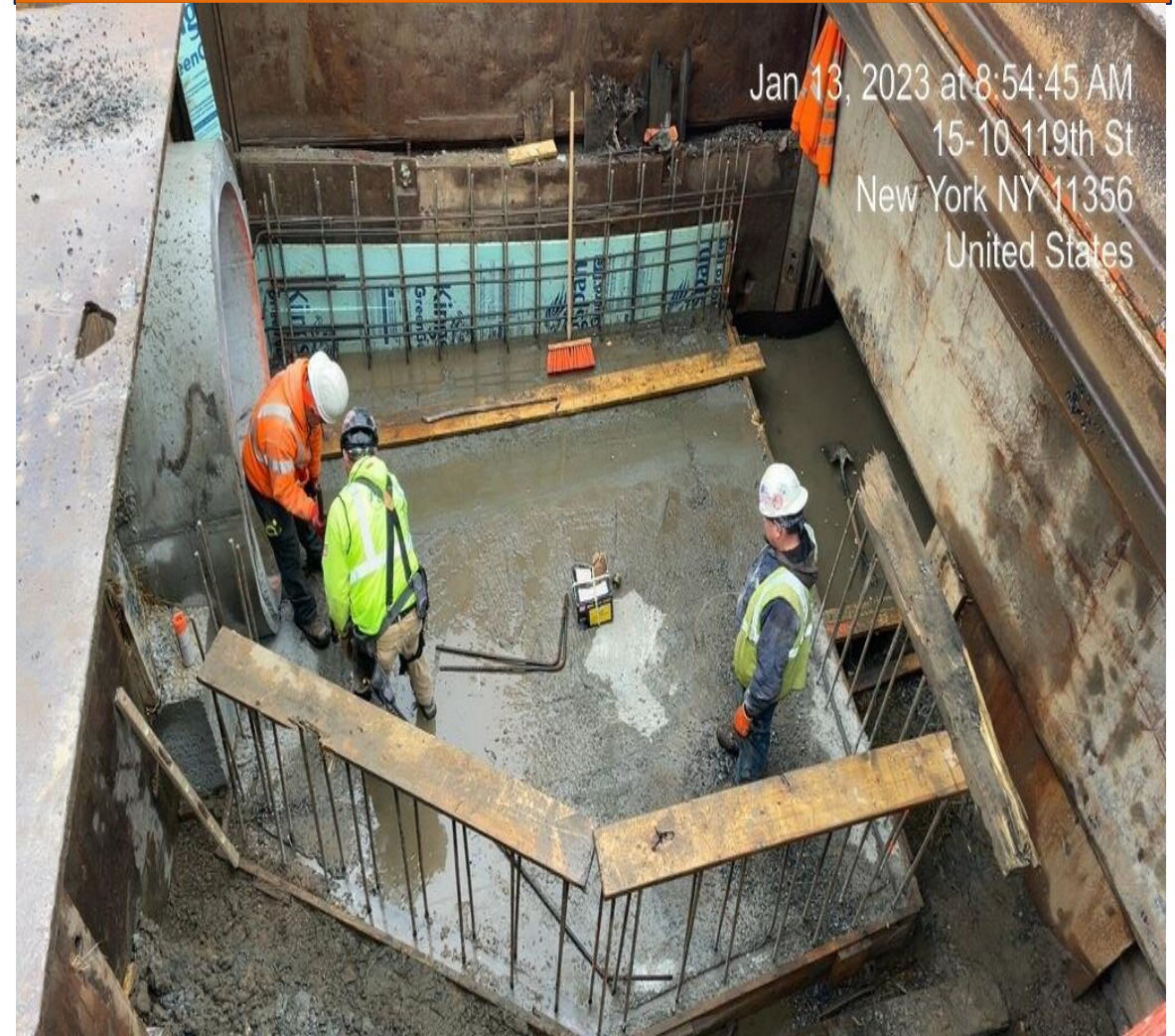
Chamber No. 2 Intersection of 15 th Avenue and 118 th Street
