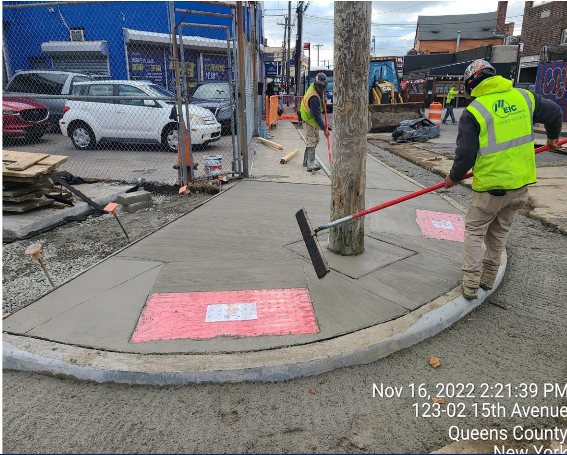
LOCATION: Intersection of 15 th Ave and 123 rd street
