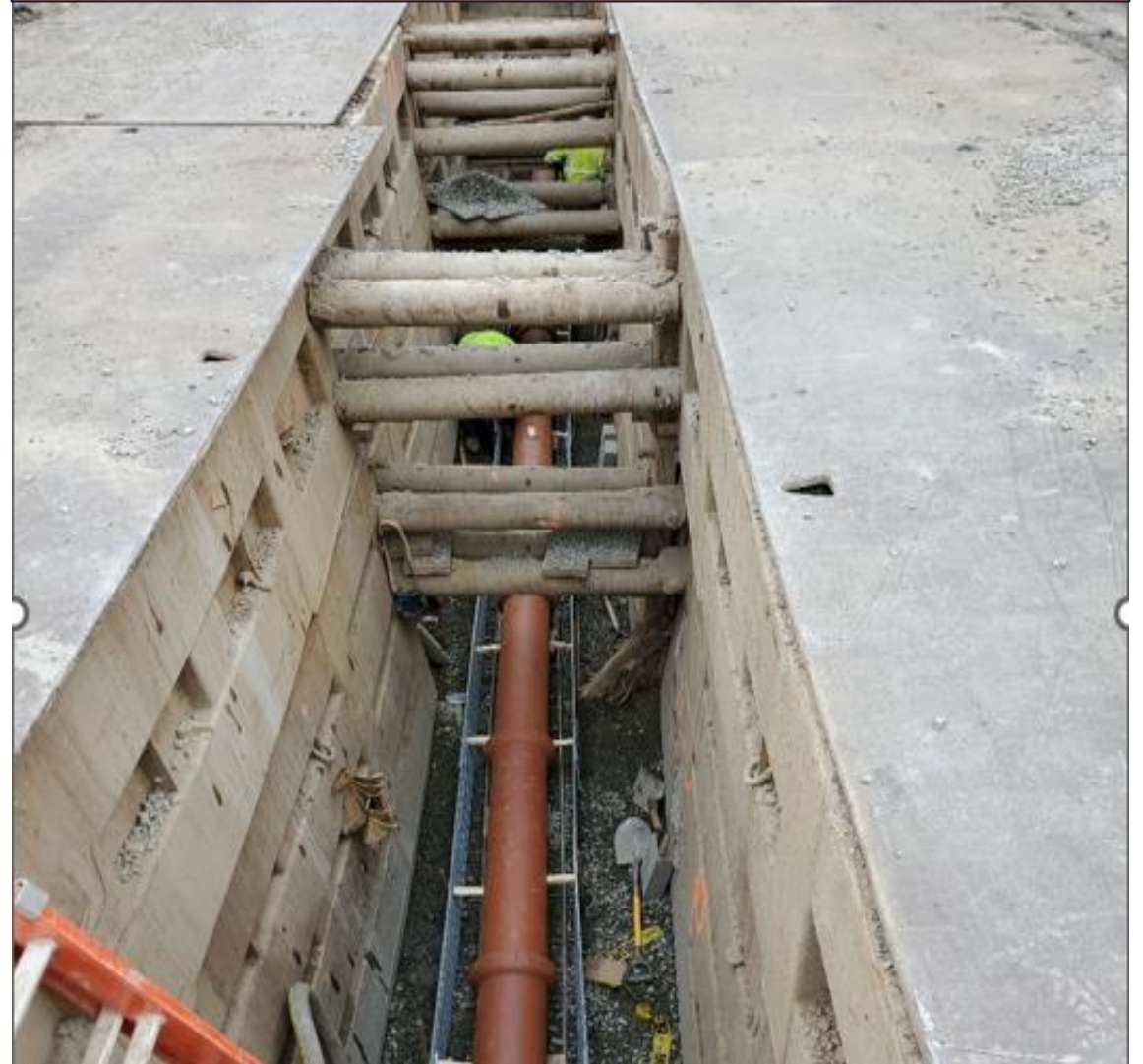
Sanitary Sewer 124 Street btw 18 Avenue – 20 Avenue
