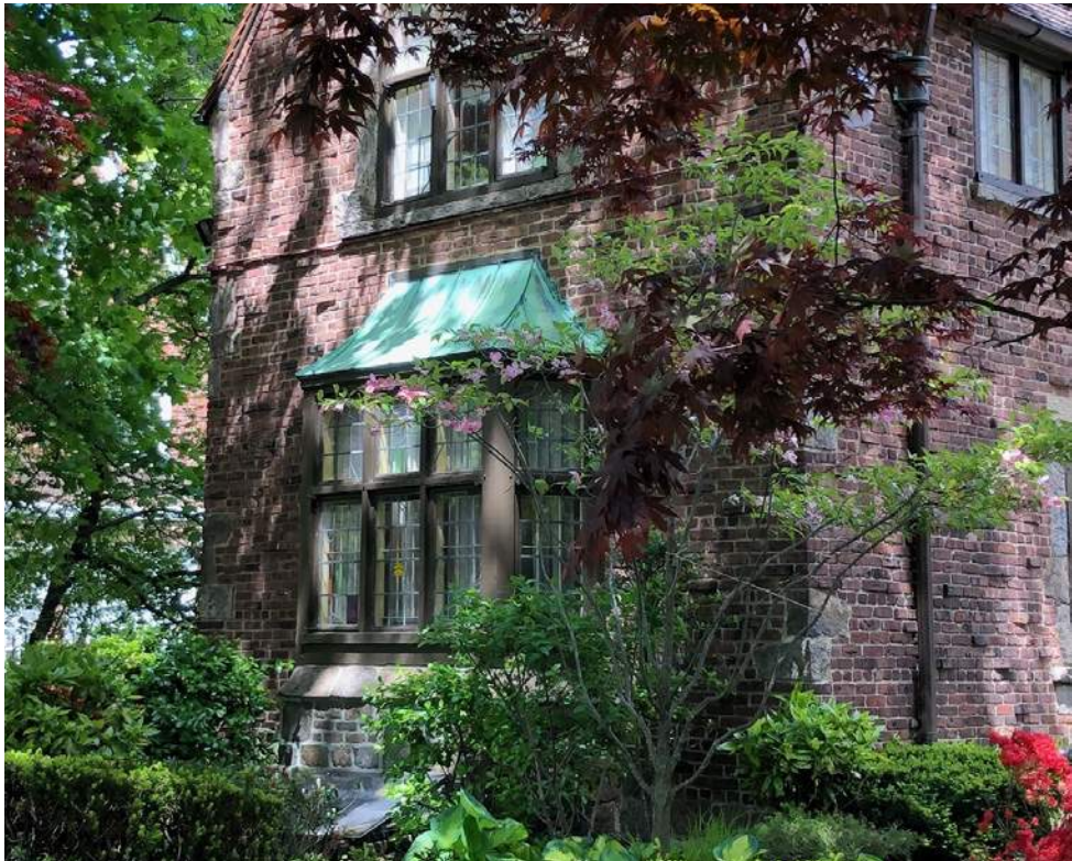
TYPICAL COPPER (OXIDIZED) DETAILS, REGO PARK
