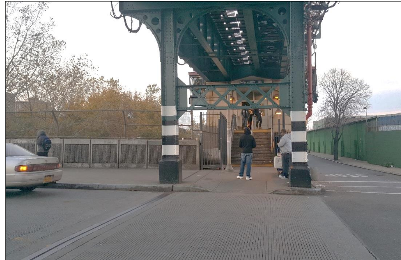
#8 View of NW Corner at Sutter Avenue and Van Sinderen Avenue, entrance to Sutter Avenue L Station.
