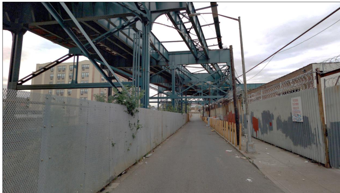
#2 Van Sinderen Avenue under the Elevated L line between Liberty Avenue and Pitkin Avenue.
