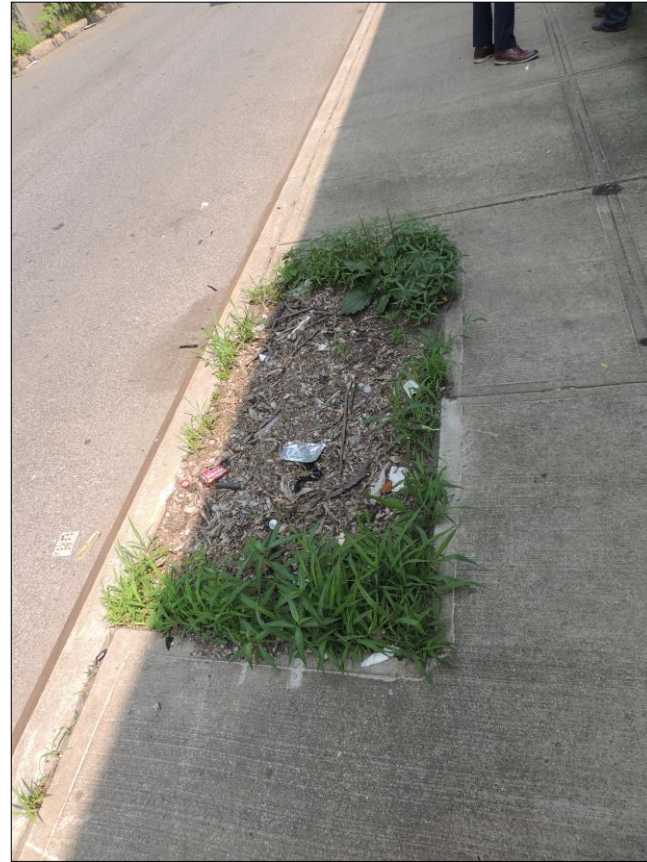
#7 Existing tree pit located along Van Sinderen Avenue near Sutter Avenue intersection.
