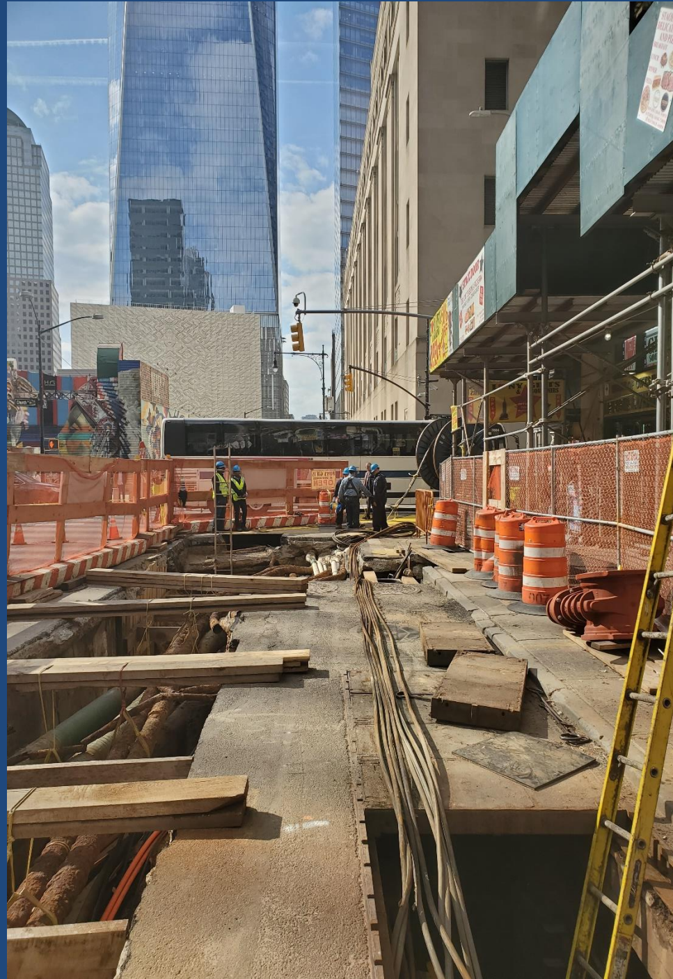
Removal of Electrical Cables
