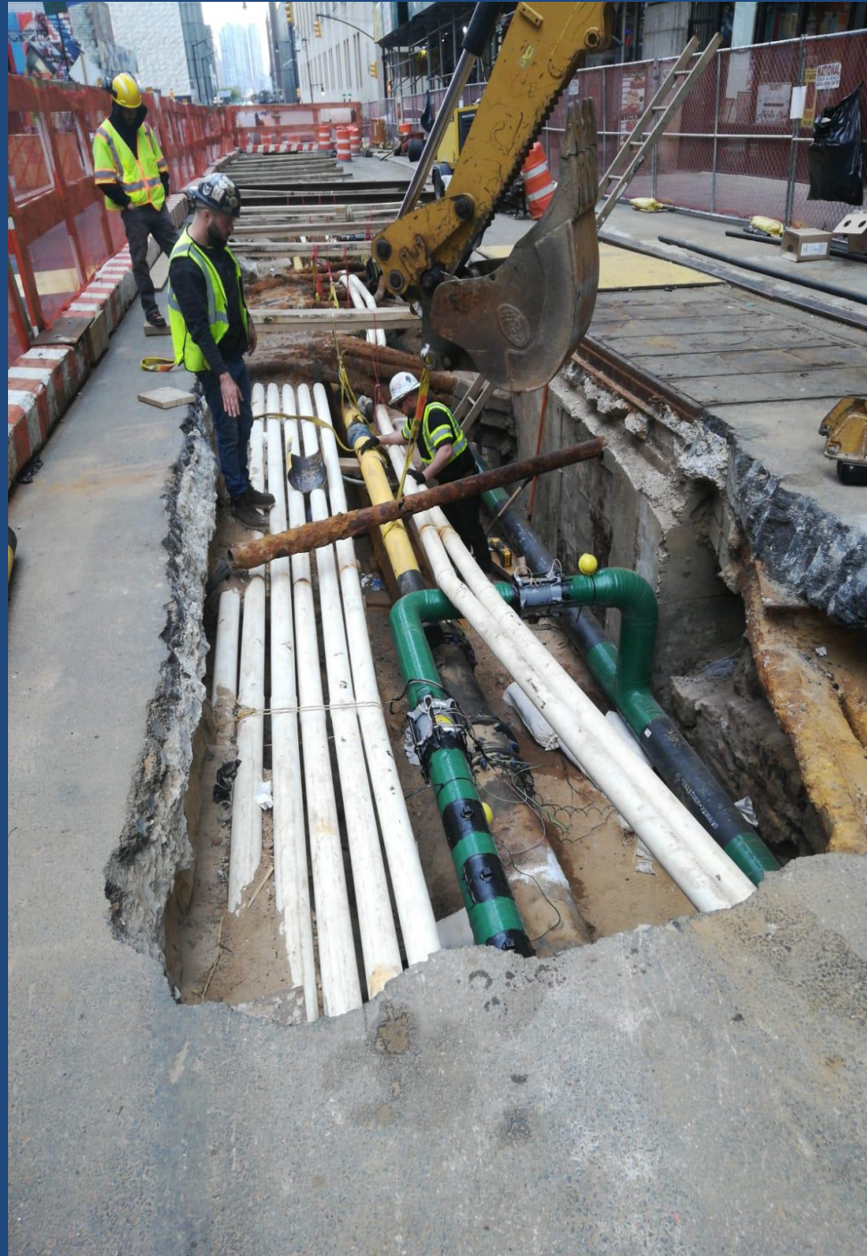
Installation of 8" Steel Gas
