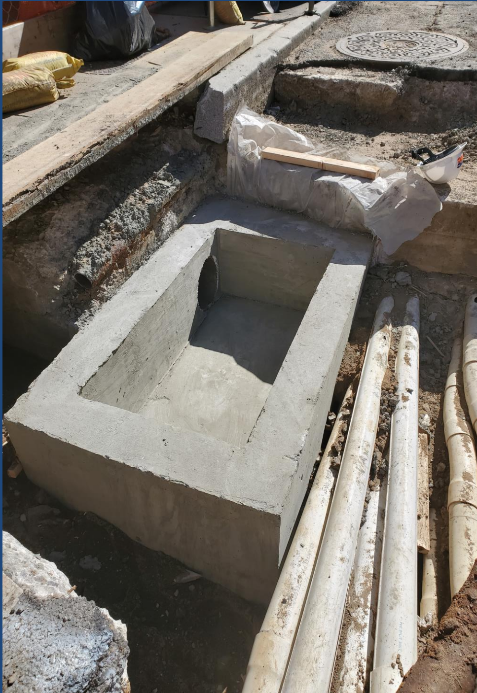
Cast in Place Catch Basin
