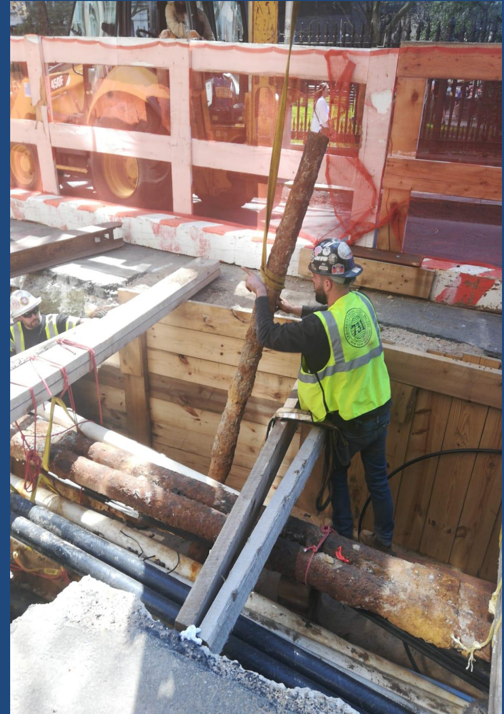
Removal of 4" Electric Conduits
