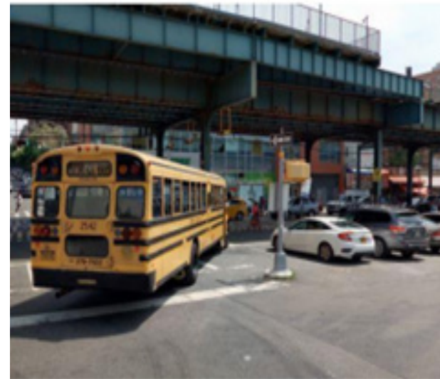
Unclear demarcations (Elliot Place)
