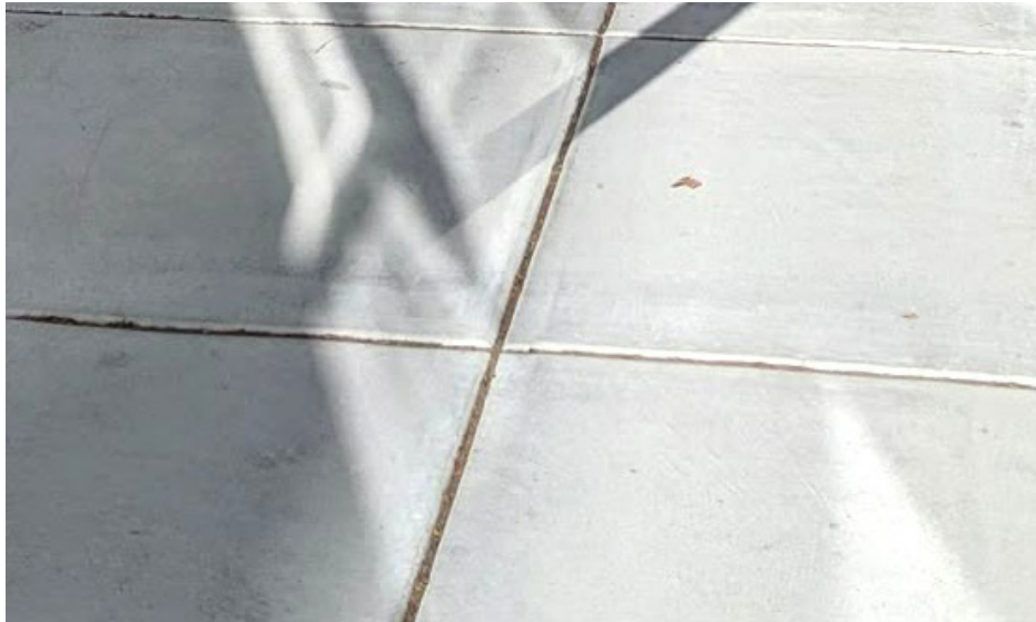
Typical Sidewalk Concrete
