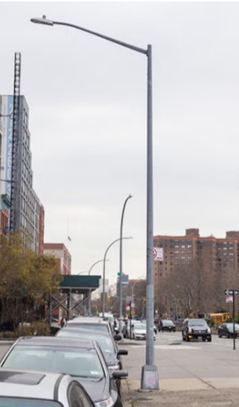
Octagonal Pole and Cobra Head Luminaire
