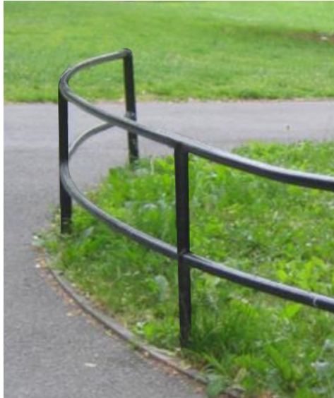
Type "B" Pipe Rail Fence
