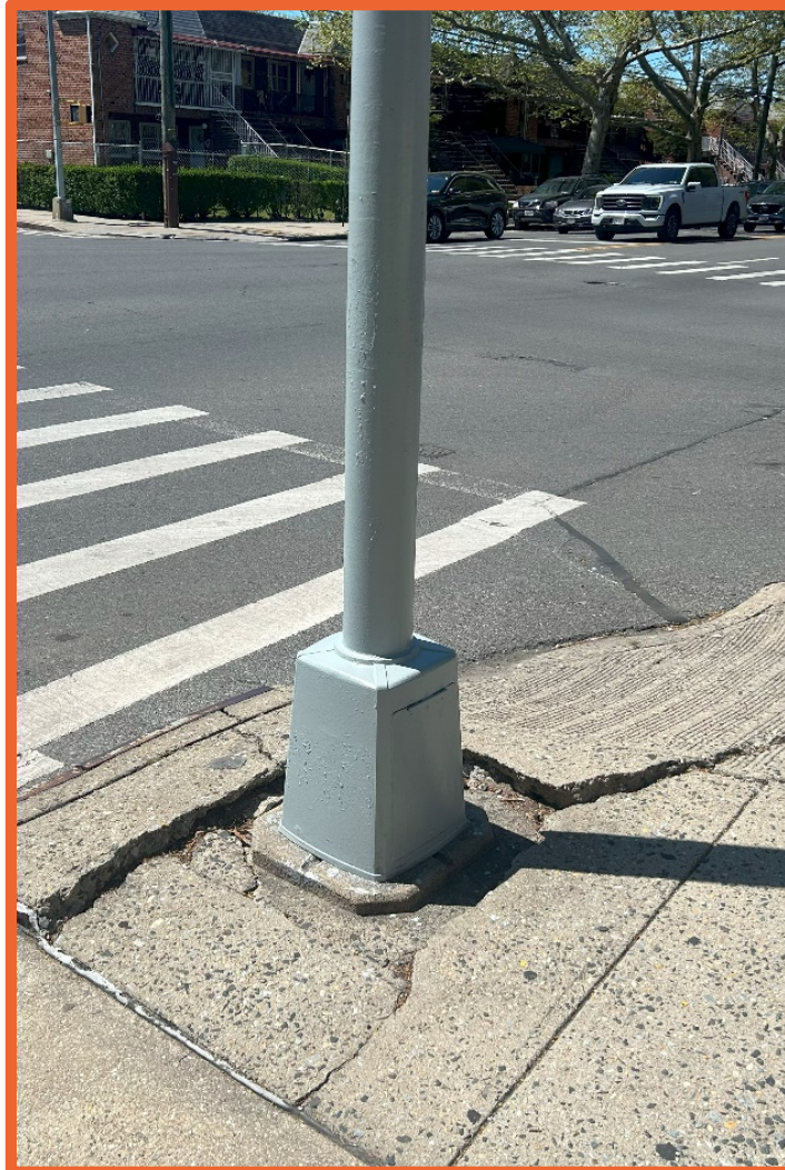
Cracked Sidewalks
