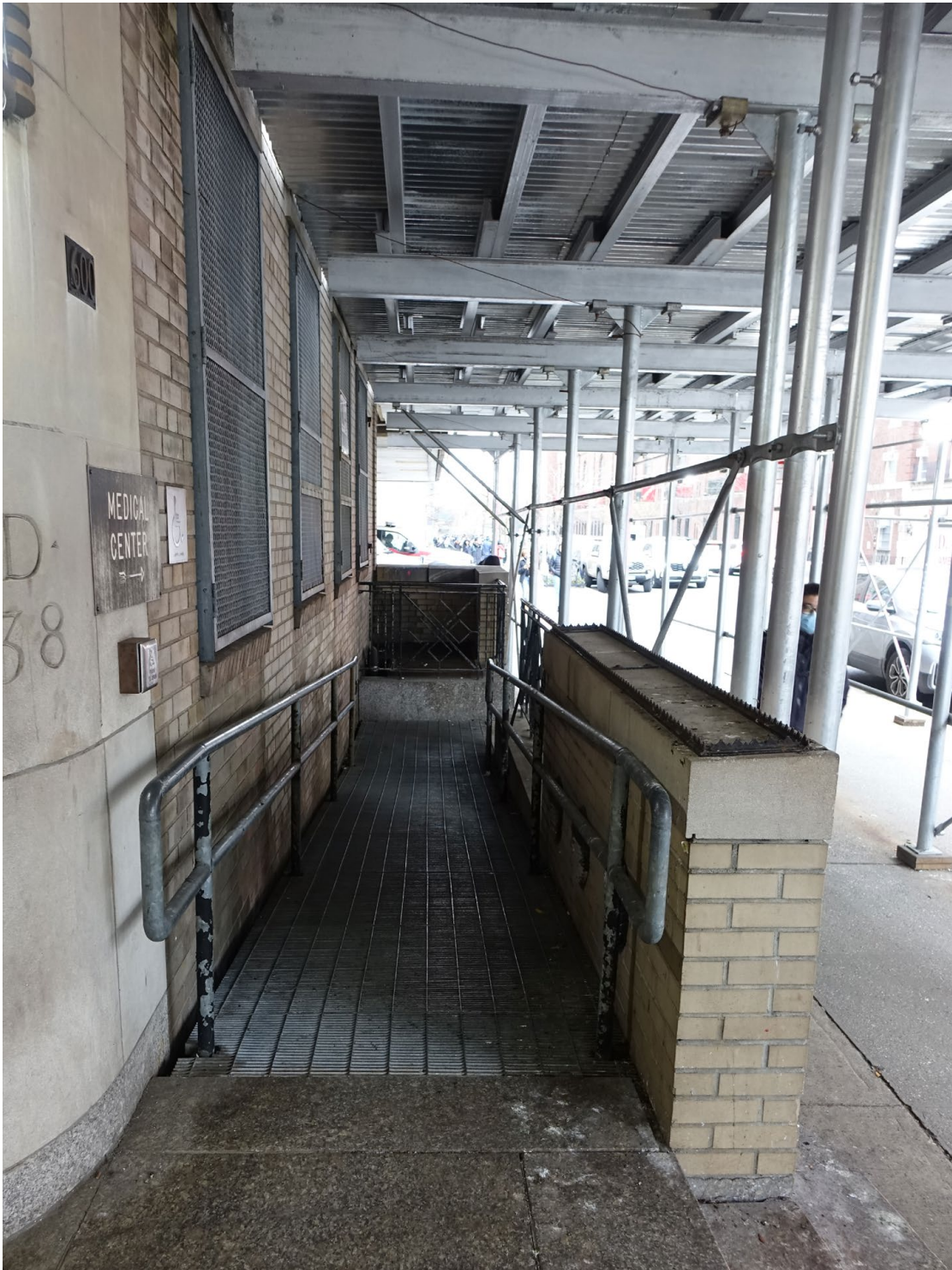
16._ EXISTING RAMP LANDING
