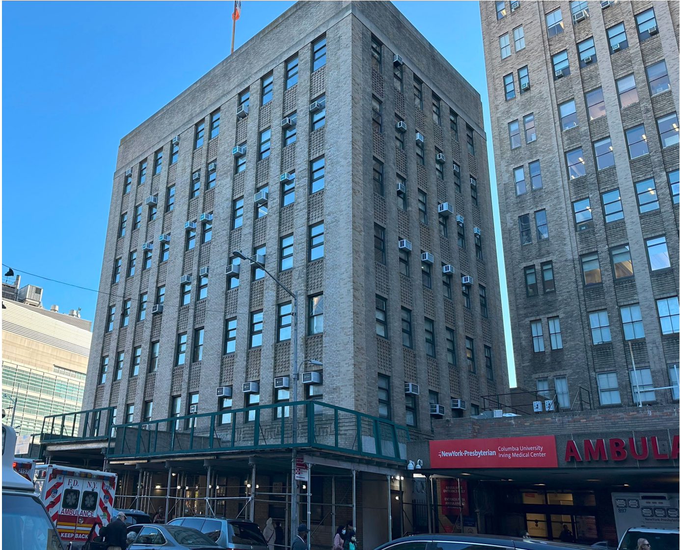
2._ NORTH WEST VIEW FROM SIDEWALK ALONG 168TH ST.
