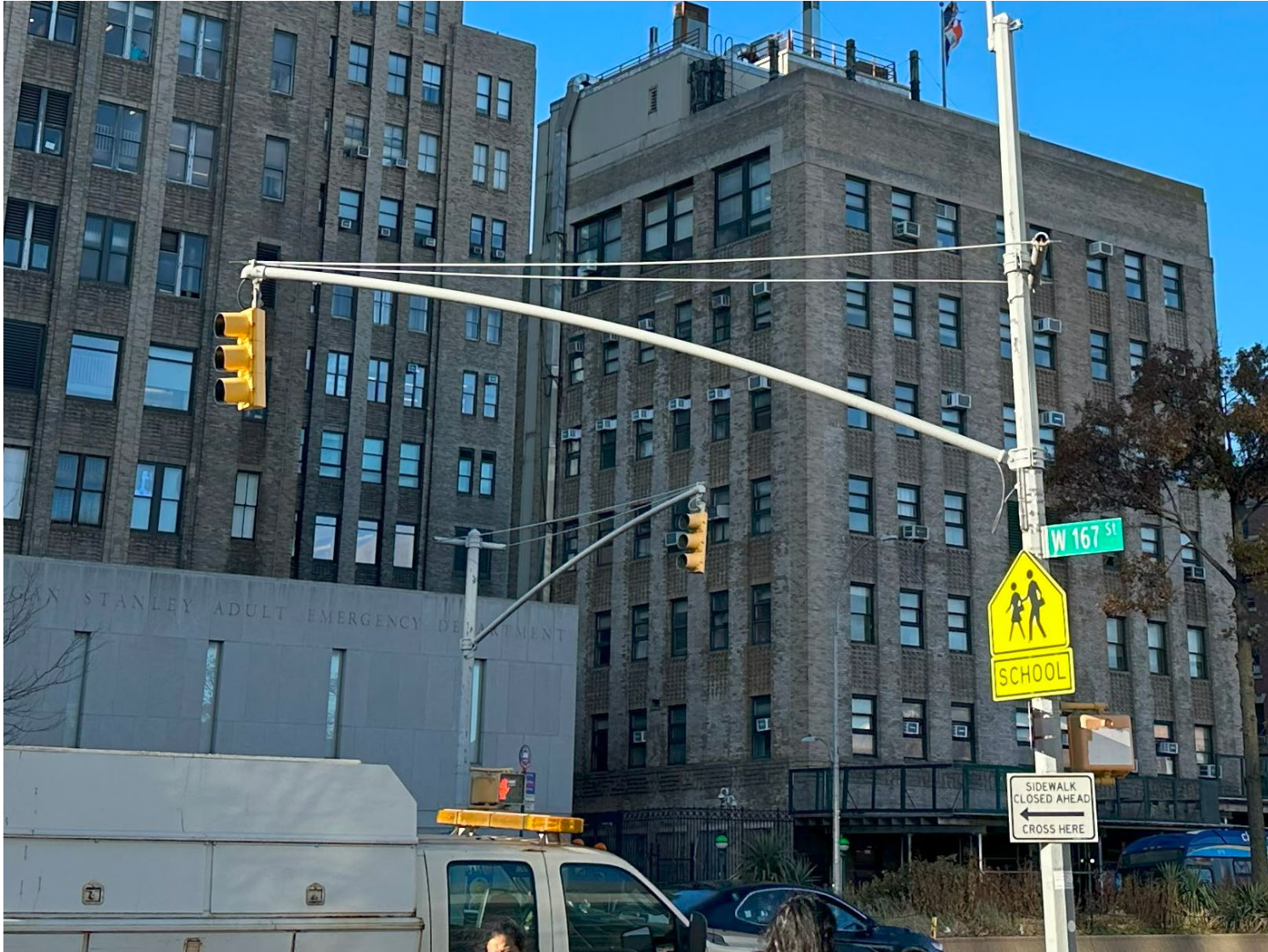
1._ SOUTH EAST VIEW FROM SIDEWALK CORNER ALONG BROADWAY
