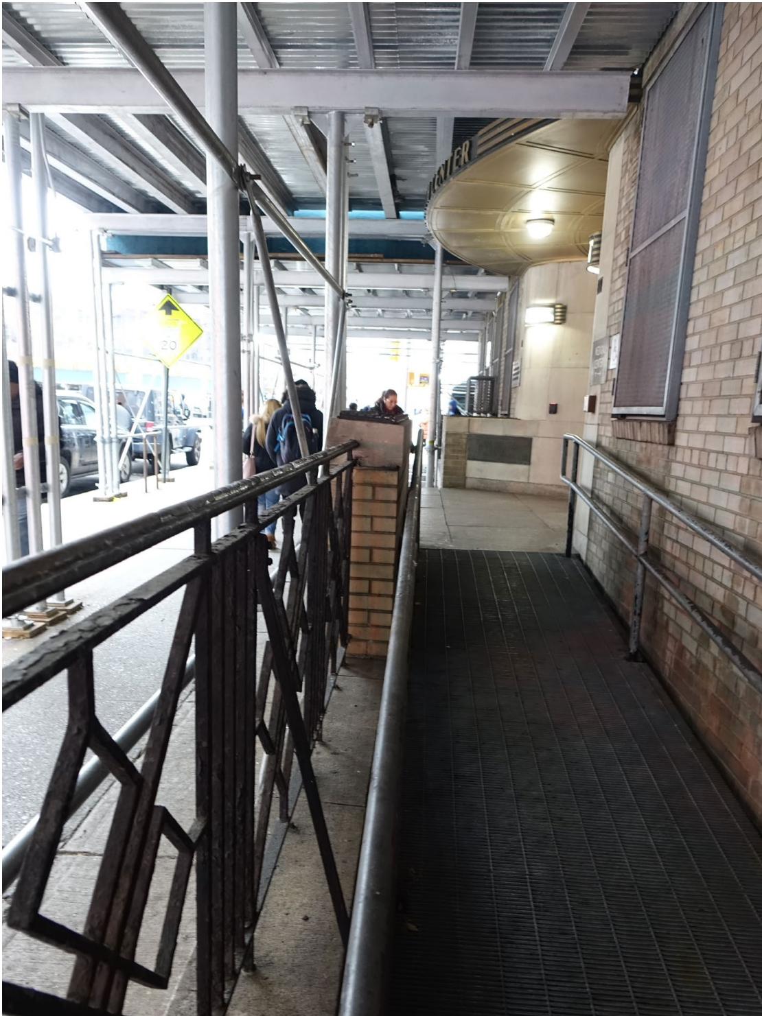
15._ EXISTING RAMP TOP LANDING
