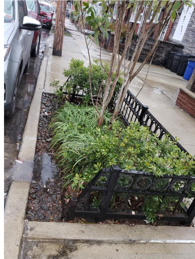
Constructed Rain Garden in Maspeth, NY
