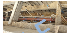
Installation of Sanitary Sewer on 119 th Ave.
