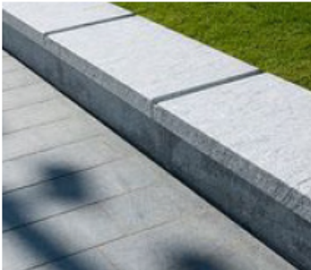
RAISED PLANTER/ SKATE STOP CONCRETE WITH NOTCHES
