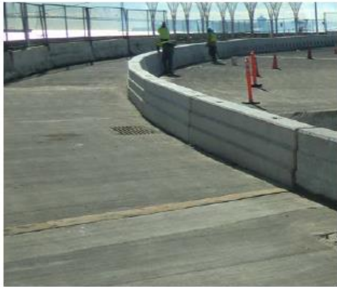
BICYCLE BARRIER WALL
